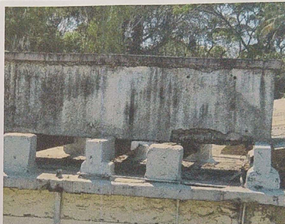
Spalling off concrete and Exposed corroded reinforcement of water tank (not in use)
