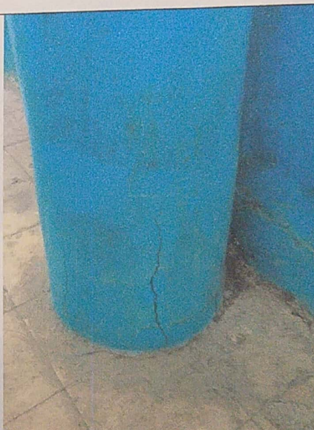
Distressed Columns on first floor near girl's toilet
