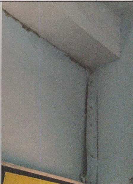
Open construction joint
