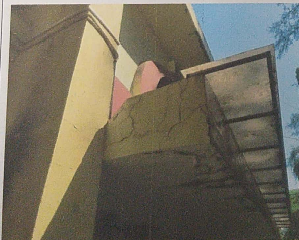
Cracks in the slab of the entrance porch
