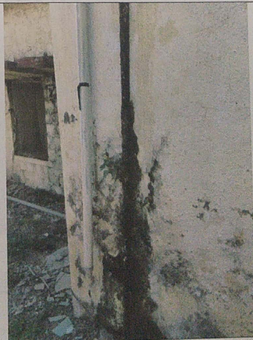
Vegetative growth and leakages through plumbing lines
