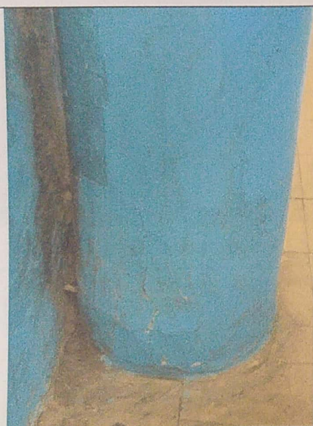
Distressed Columns on first floor near girl's toilet
