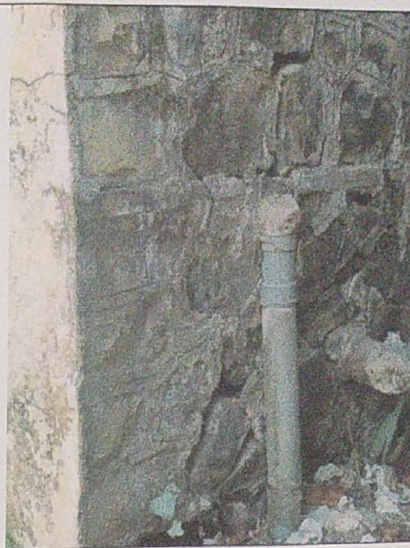
Masonry cracks in exterior face of wall
