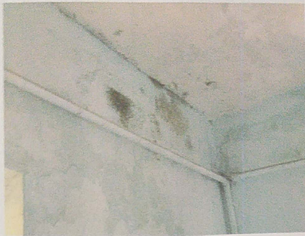
Seepage in toilet of primary section
