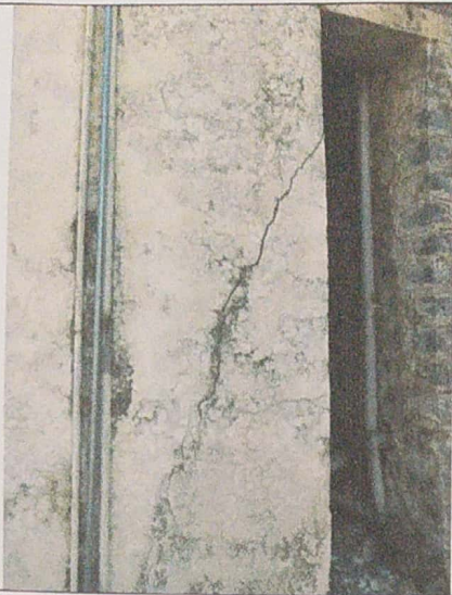
Masonry crack in exterior face of wall
