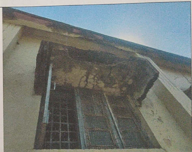
Broken chajja with spalling off concrete and exposed corroded reinforcement
