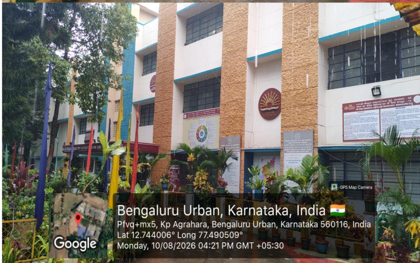
FIG. NO. 3& FIG. NO. 4: GENERAL SIDE VIEW OF PM SHRI KENDRIYA VIDYALAYA, MG RAILWAY COLONY BENGALURU, 560023
