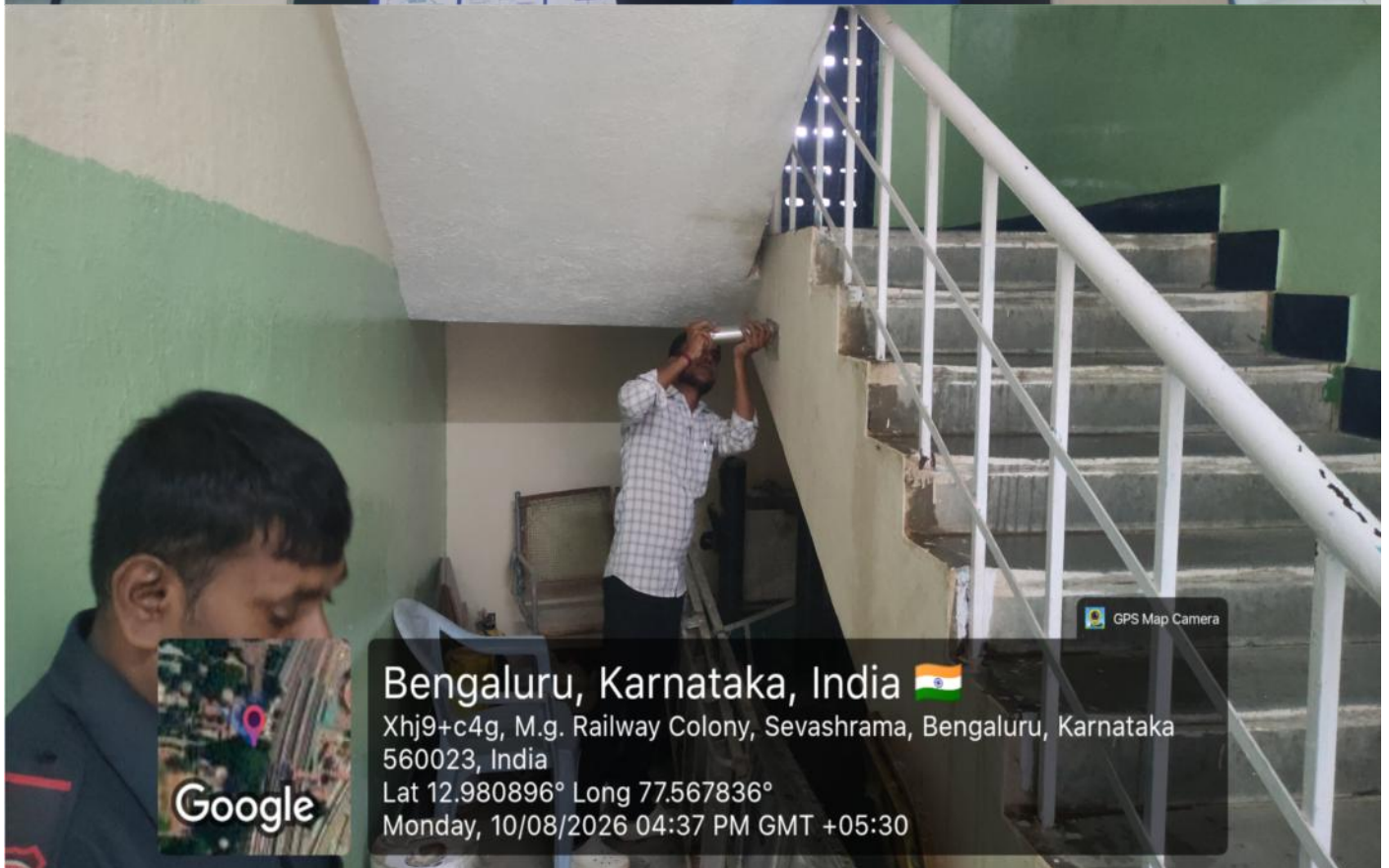
FIG. NO. 11& FIG.NO. 12: REBOUND HAMMER TEST AT SELECTED BEAM PM SHRI KENDRIYA VIDYALAYA, MG RAILWAY COLONY BENGALURU, 560023
