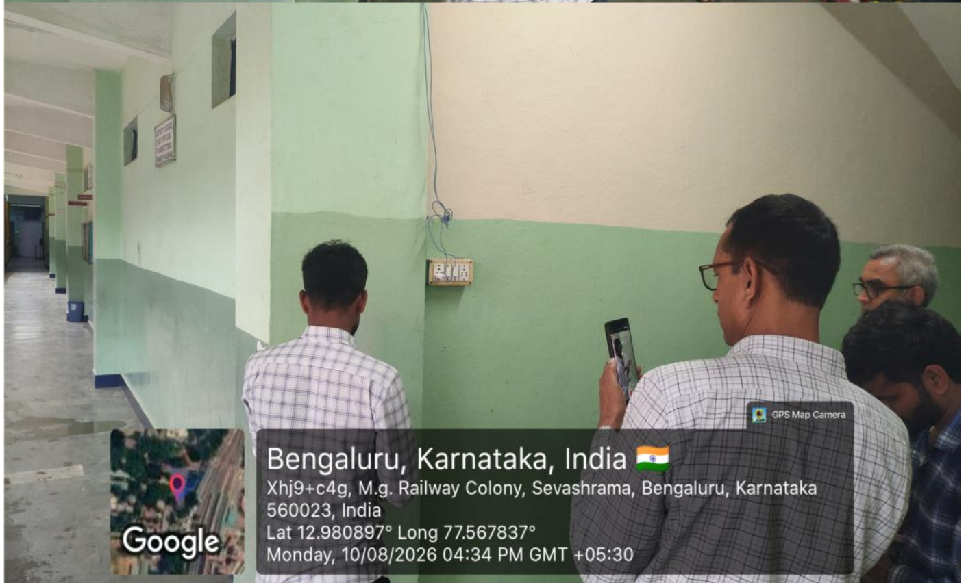
FIG. NO. 9& FIG.NO. 10: REBOUND HAMMER TEST AT SELECTED COLUMN PM SHRI KENDRIYA VIDYALAYA, MG RAILWAY COLONY BENGALURU, 560023
