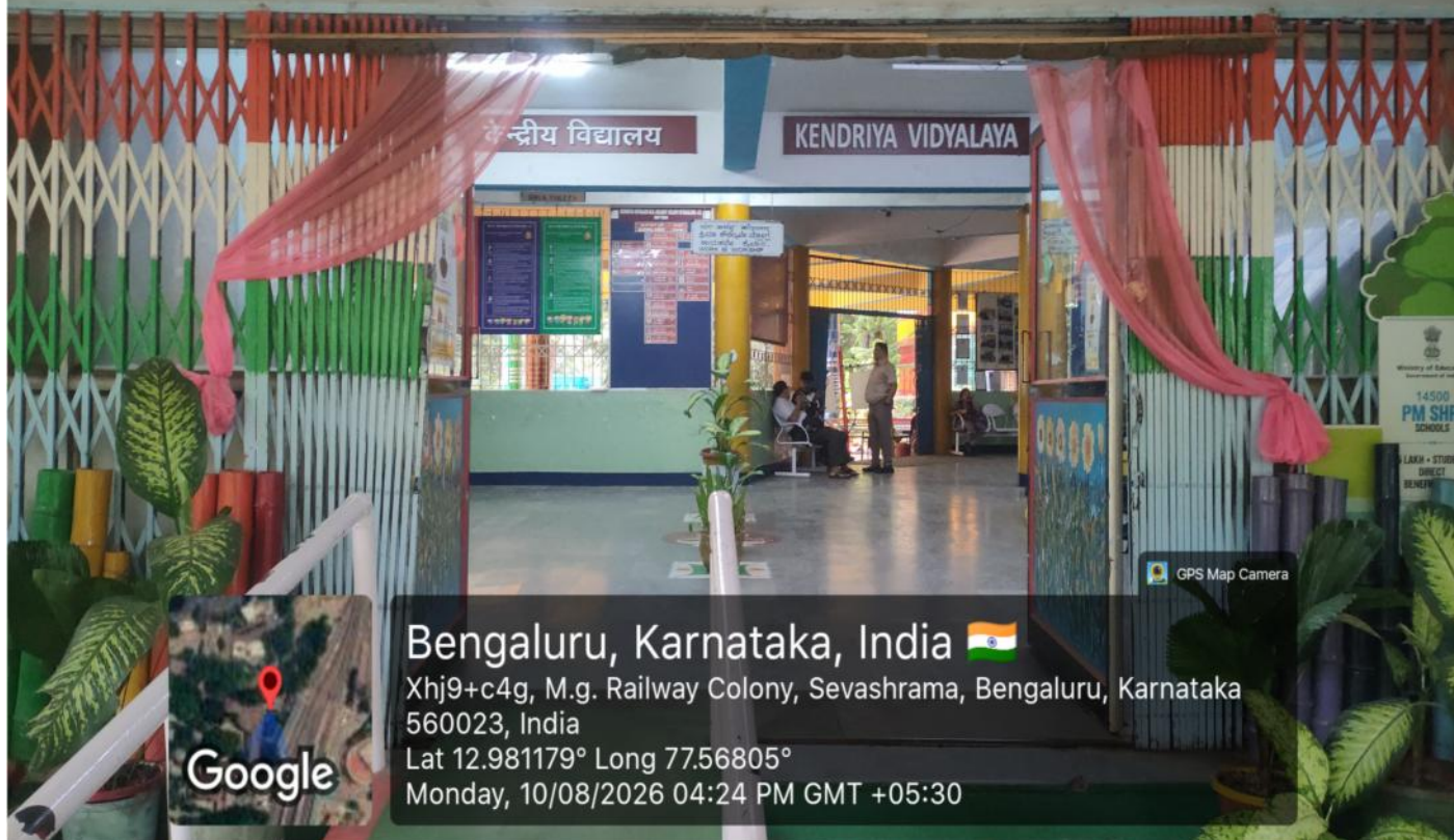
FIG.NO. 5& FIG. NO. 6: GENERAL CORRIDOR AND FRONT VIEWS AT PM SHRI KENDRIYA VIDYALAYA, MG RAILWAY COLONY BENGALURU, 560023
