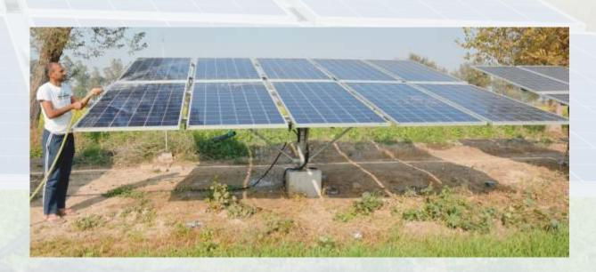
Daily switch on the pump in the morning at around 7.00 AM (sooner the better) and switch off in the evening after 5.30PM. Switch is provided on the controller. Installation team will provide training on how to switch on and off the pump.
