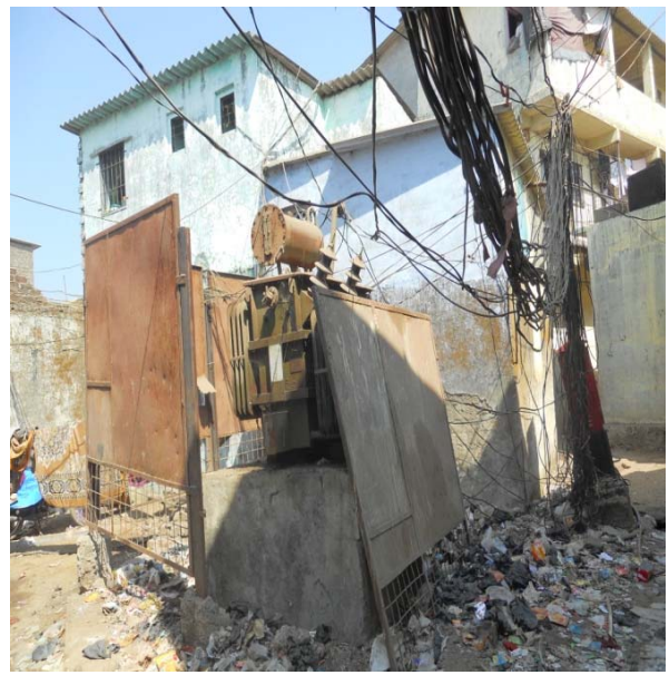
Above left: Tapped electric connections in Rashid Compound, ward no.114. Open transformer which poses a threat to the residents in the area. Above right: Tapped electric connection in Rashid Compound, ward no. 114.
