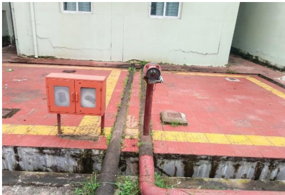
(HOSE REEL AND HYDRANT SYSTEM)
