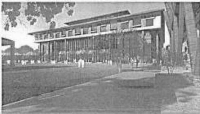
Srinagar District Court
