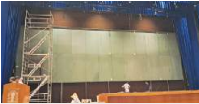
Installation of Video Wall in Auditorium, C block, Additional Building Complex
