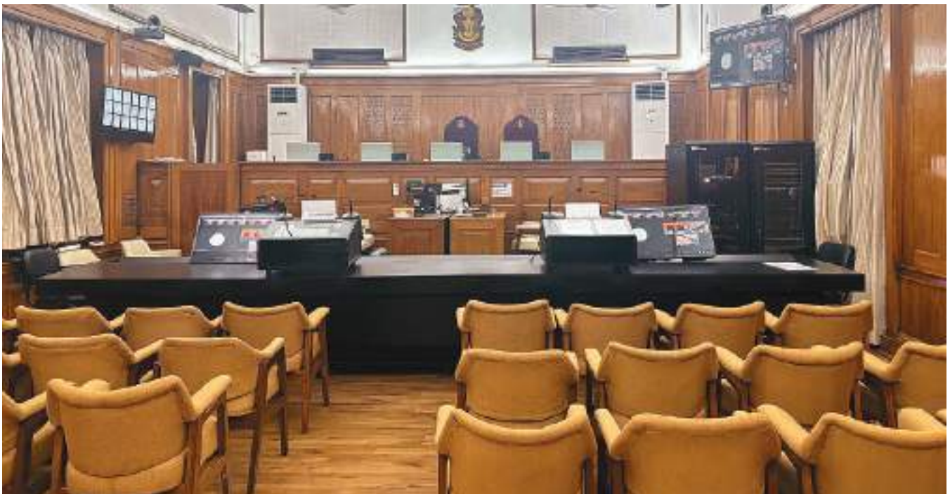
Courtroom No 3 after renovation being made apt for the futuristic and technologically advanced infrastructure during summer vacation 2024, Main Campus, Supreme Court of India
