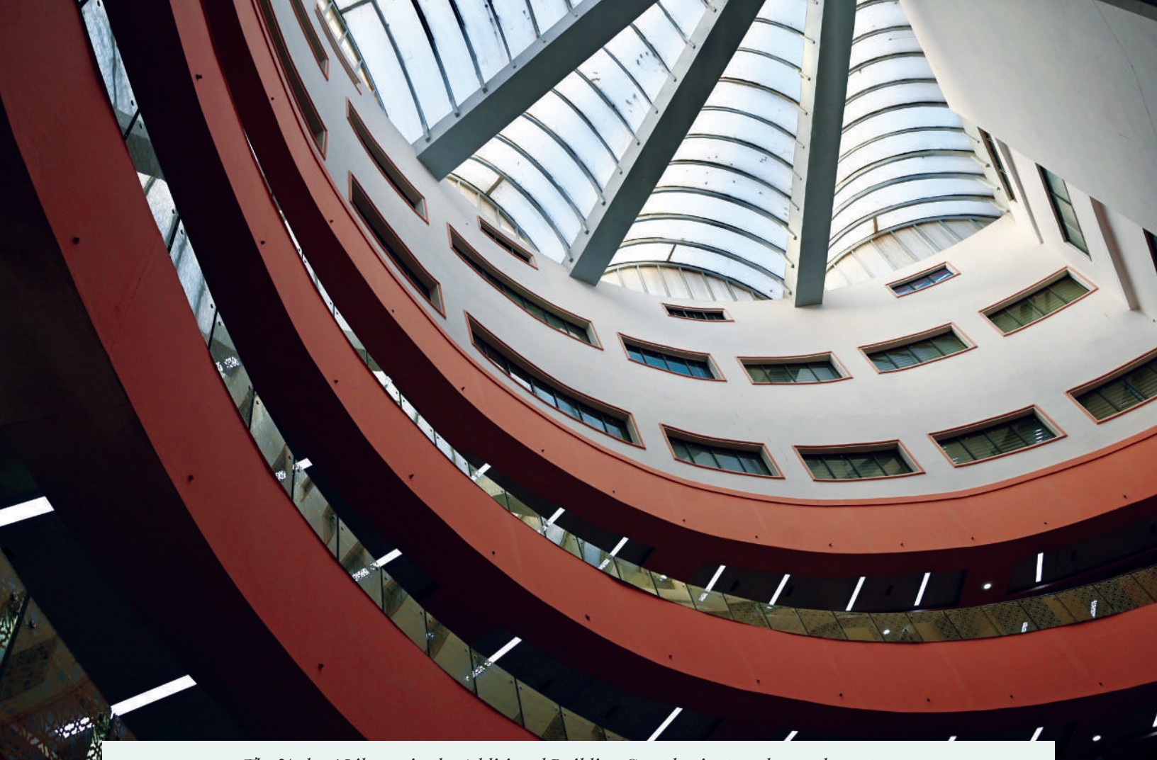
The Judges' Library in the Additional Building Complex is spread over three storeys
