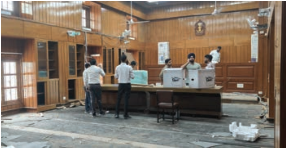
Courtroom no 6 among other courtrooms including 7, 8, and 9 being renovated to make them futuristic and technologically advanced during vacation
