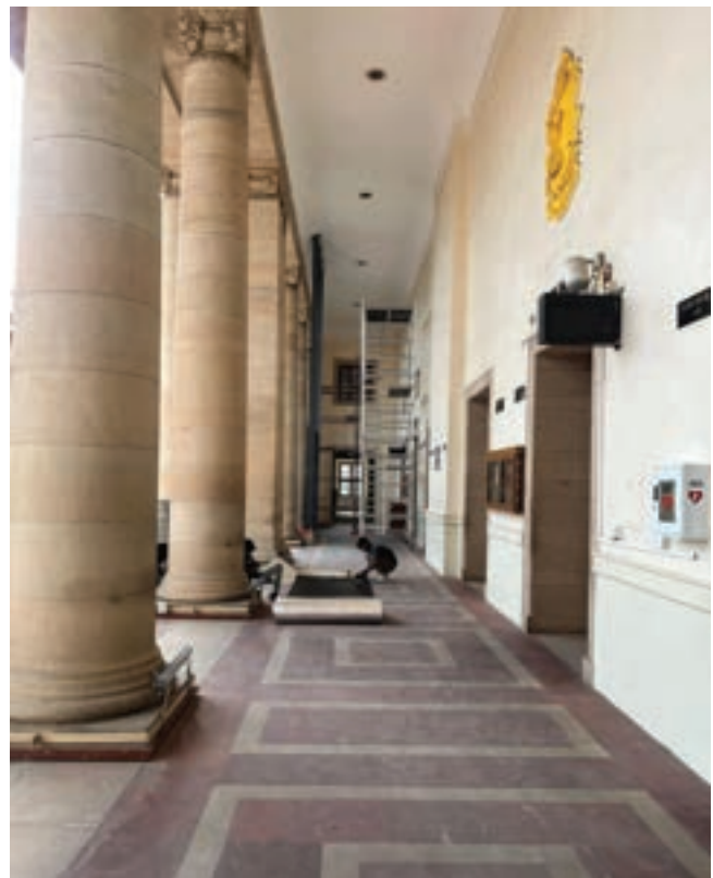
Ongoing repairs at Supreme Court during summer vacation
