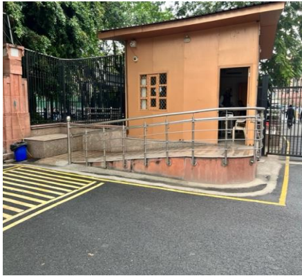
Accessible entrance with adequate space for alighting from vehicle
