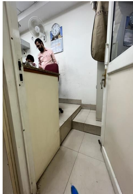
Ramps required, due to paucity of space for ramp with acceptable gradient it is suggested to relocate the office
