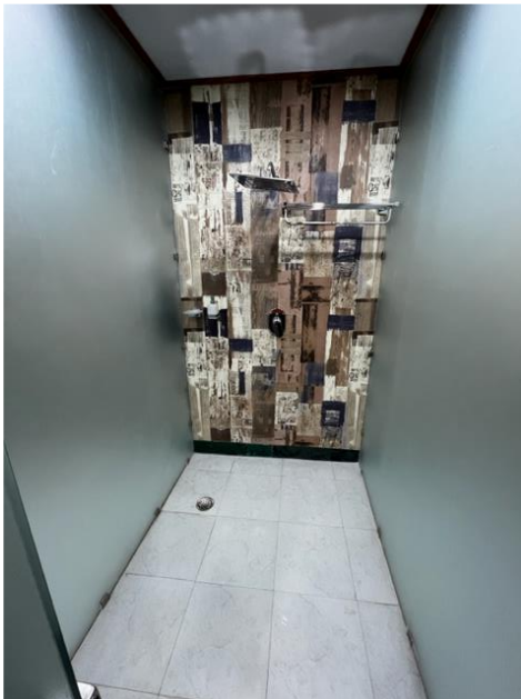
Changing cubicles have thin walls which cannot mount handrails
