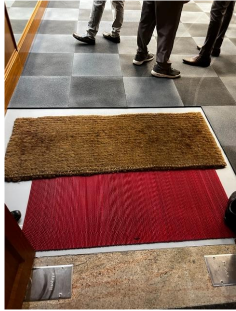
Mattress can be an impediment to small front wheel of wheelchair and a person can trip
