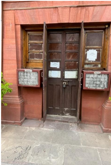
Threshold, ramp required
