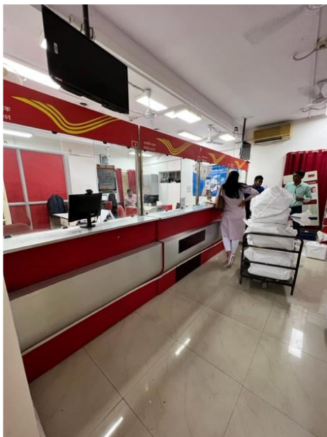
Counter too high for a wheelchair bound person to access. Threshold needs to be levelled, a trip hazard and an impediment for wheelchair user
