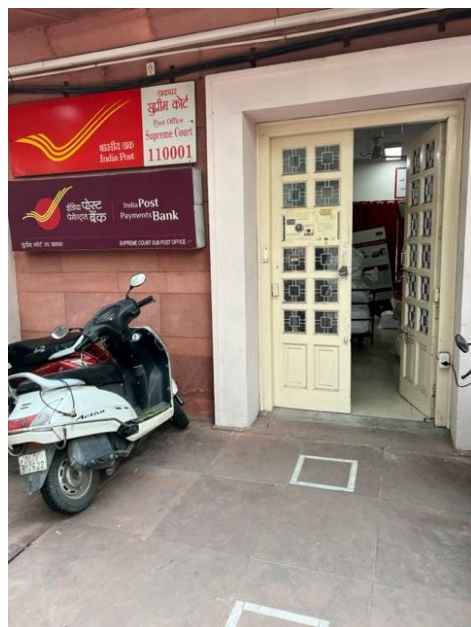
Counter too high for a wheelchair bound person to access. Threshold needs to be levelled, a trip hazard and an impediment for wheelchair user
