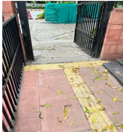
Tactile Tiles covered by leaves, need regular cleaning
