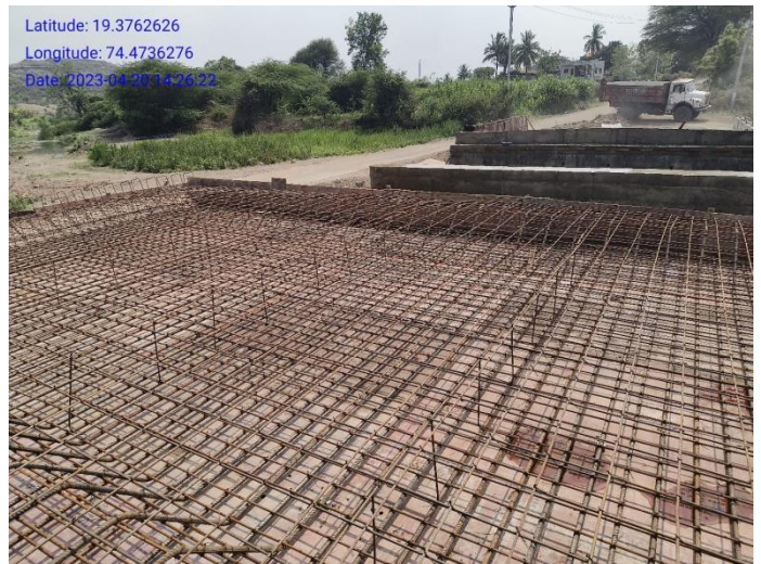
Slab Reinforcement
