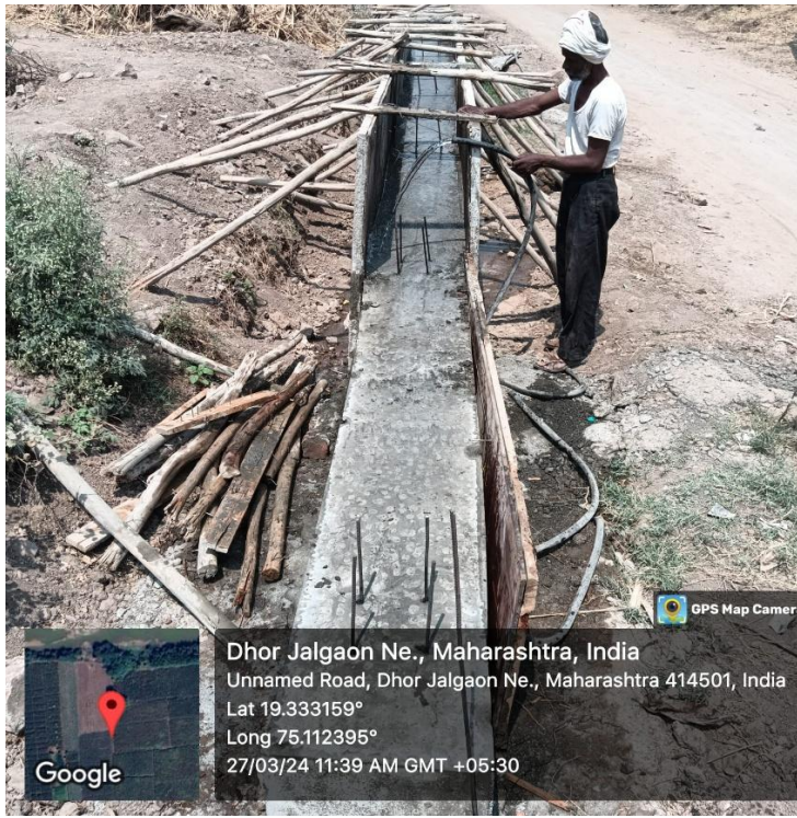
Construction of Protection Wall
