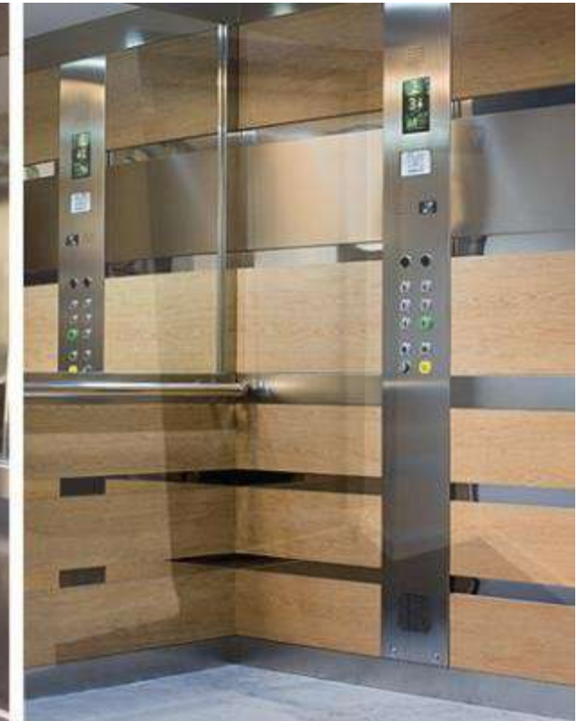
Good Practice, Bespoke lifts in UK
