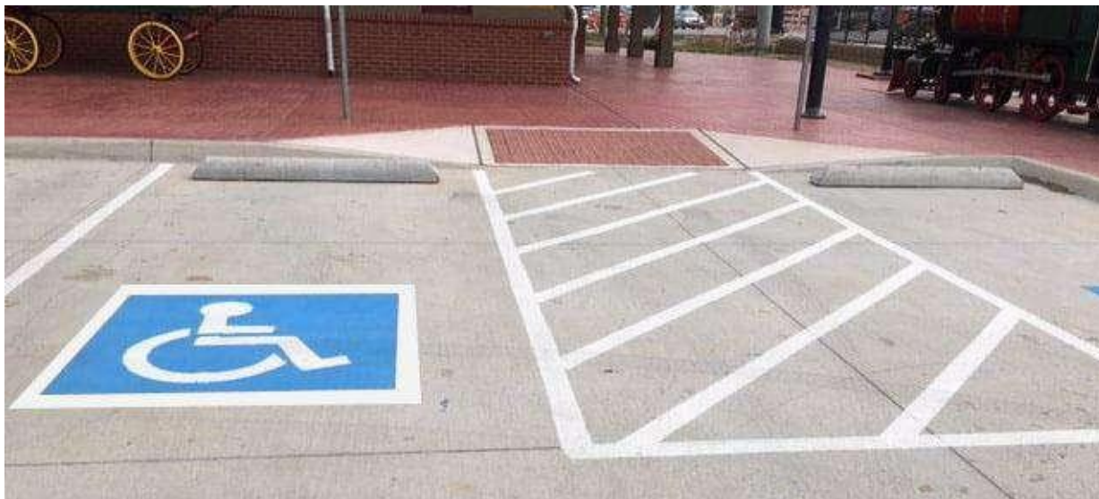
Example of parking symbol on floor, transfer bay marking and kerb ramp
