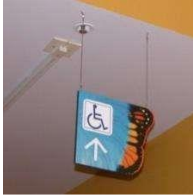
Photo 5-3. Ceiling Hung Directional Sign
