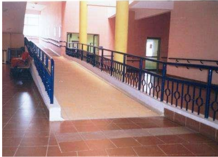
Photo 14-1. Ramp adequately illuminated with natural light
