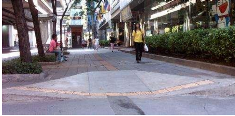
Photo 2-2. Clear and leveled approach with Kerb Ramps
