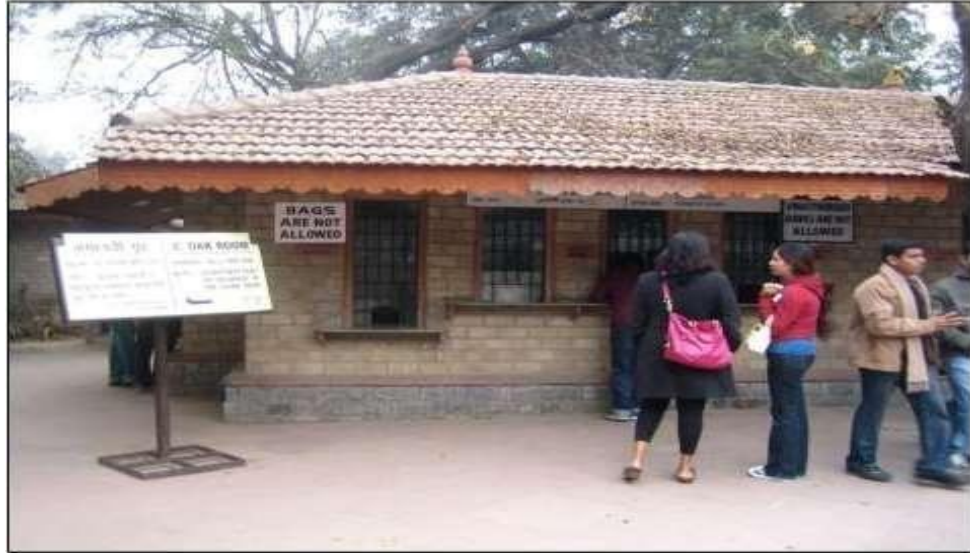
Fig 4.1: Accessible Ticket Counters at Qutub Minar Complex
