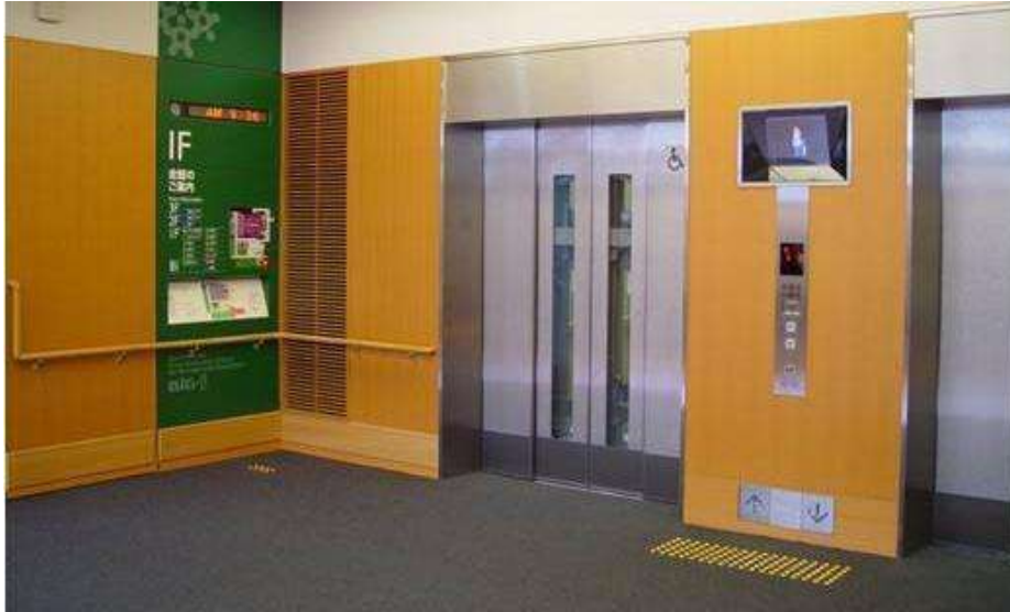
Photo 10-1. Lift signage and colour contrasted amenities
