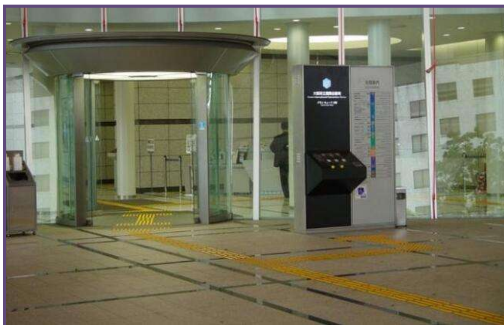
Photo 4-1. Accessible Main Entrance with Tactile Pavers
