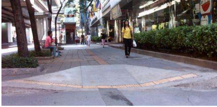
Photo 2-2. Clear and leveled approach with Kerb Ramps
