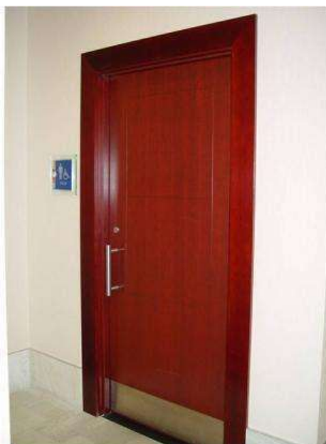
Photo 11-1. Room Signage in Braille
