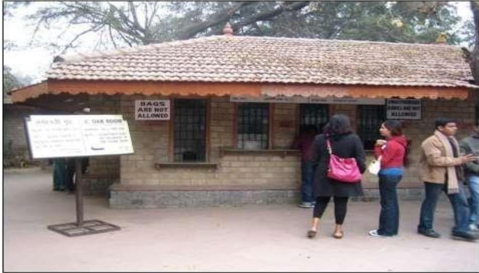
Fig 4.1: Accessible Ticket Counters at Qutub Minar Complex
