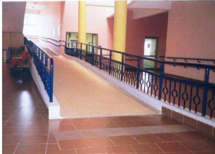
Photo 14-1. Ramp adequately illuminated with natural light
