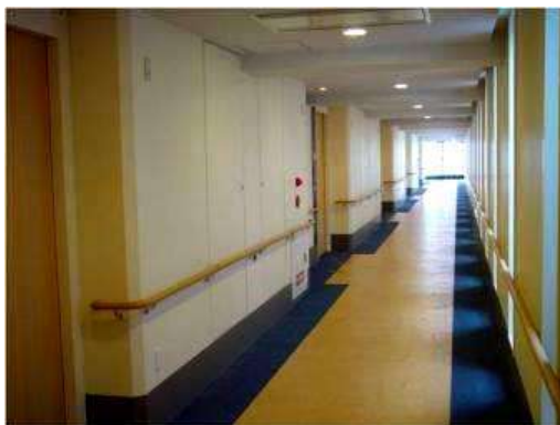
Photo 13-1. Floor finishes and visual contrast in corridor (Photo Courtesy: Joseph Kwan)
