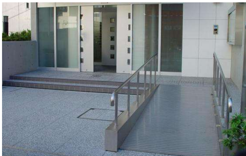
Photo 7.1 Combination of ramp and steps
