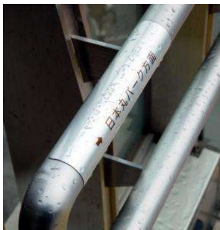
Photo 9-1. Handrail with Braille Information
