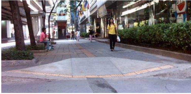
Photo 2-2. Clear and leveled approach with Kerb Ramps
