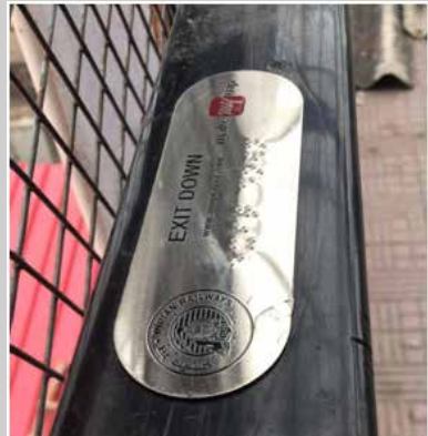
Braille Tactile Maps and Braille Indicators/Signage provided along the handrail, for ease of navigation in Dehradun Railway Station
