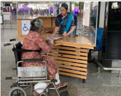
Low height counters for wheelchair users in Netaji Subhash Chandra Bose International Airport, Kolkata
