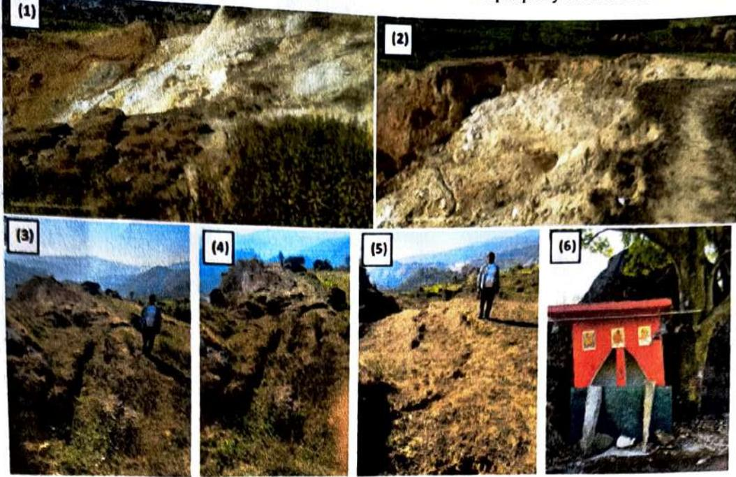
**Naveen Kumar Mines:** Field photographs showing debris slides in the dump material and ground cracks in the periphery of the mine.
