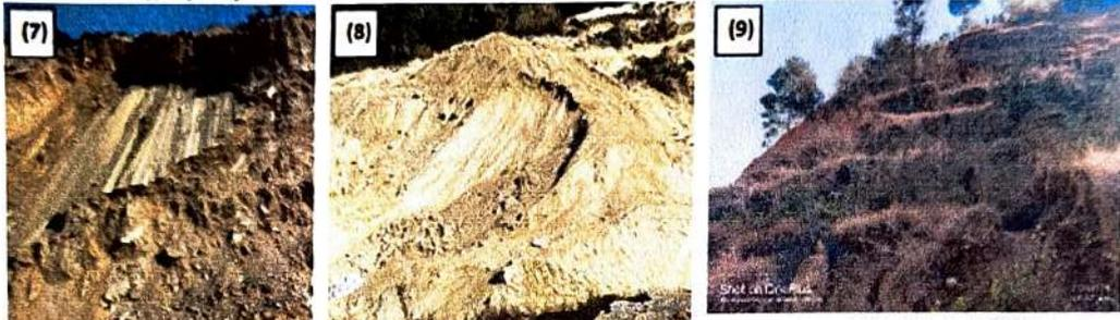
**NS Mines:** Field photographs showing debris slides and ground cracks in the dump material present within the mine.
