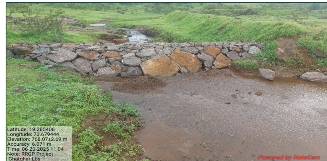
Gabion structure & loose boulder structure at intervention sites
