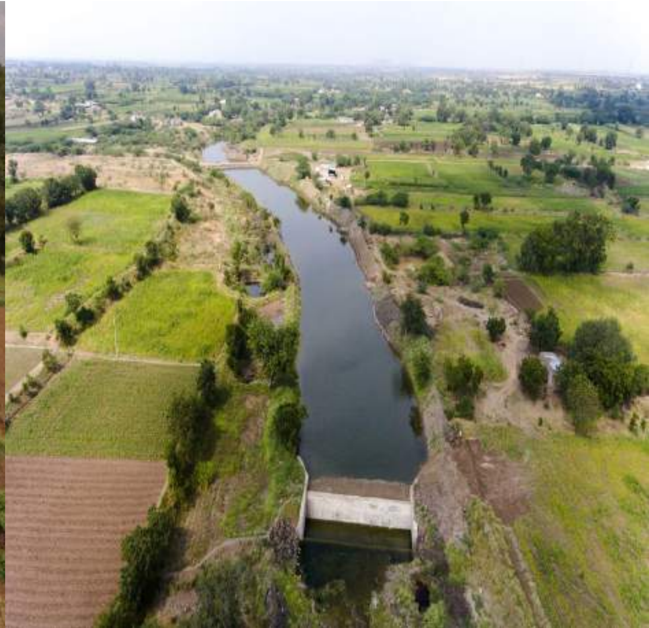
Dam Gets Filled Up After good Rains on 20/10/2018
