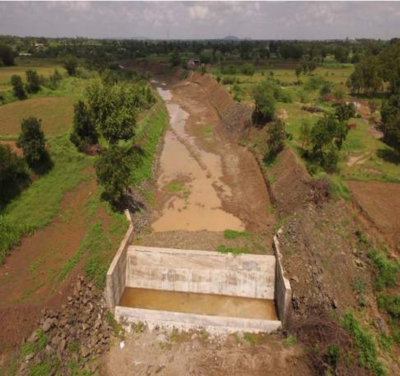
After Construction Of Check Dam Widening and Deepening of Stream Undertaken 12.08.2017
