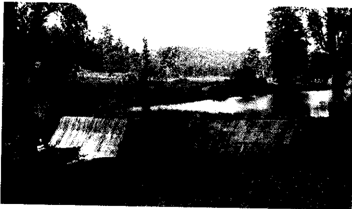
Trapping water by checkdam
