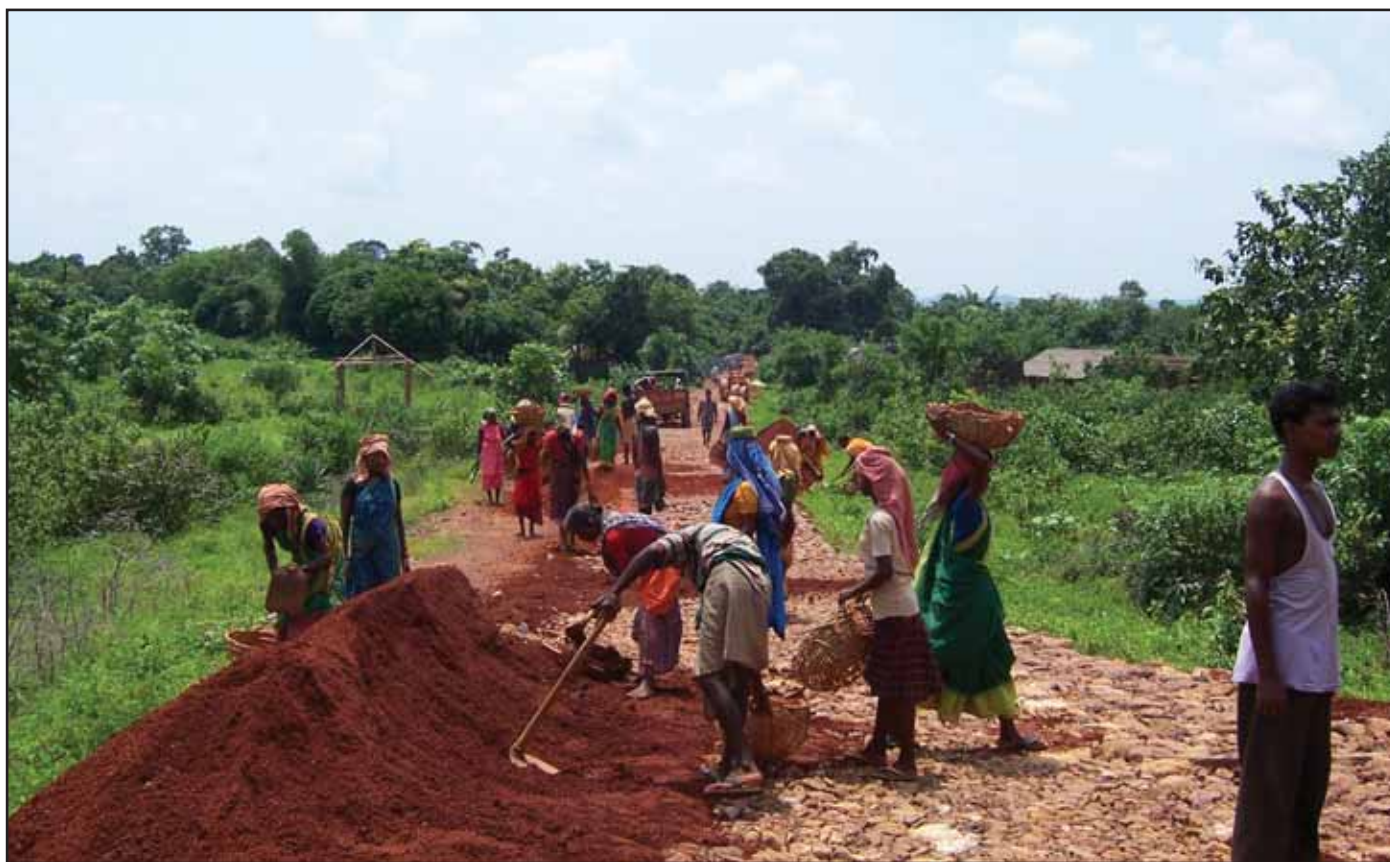
Men & Women on work under NREGA
