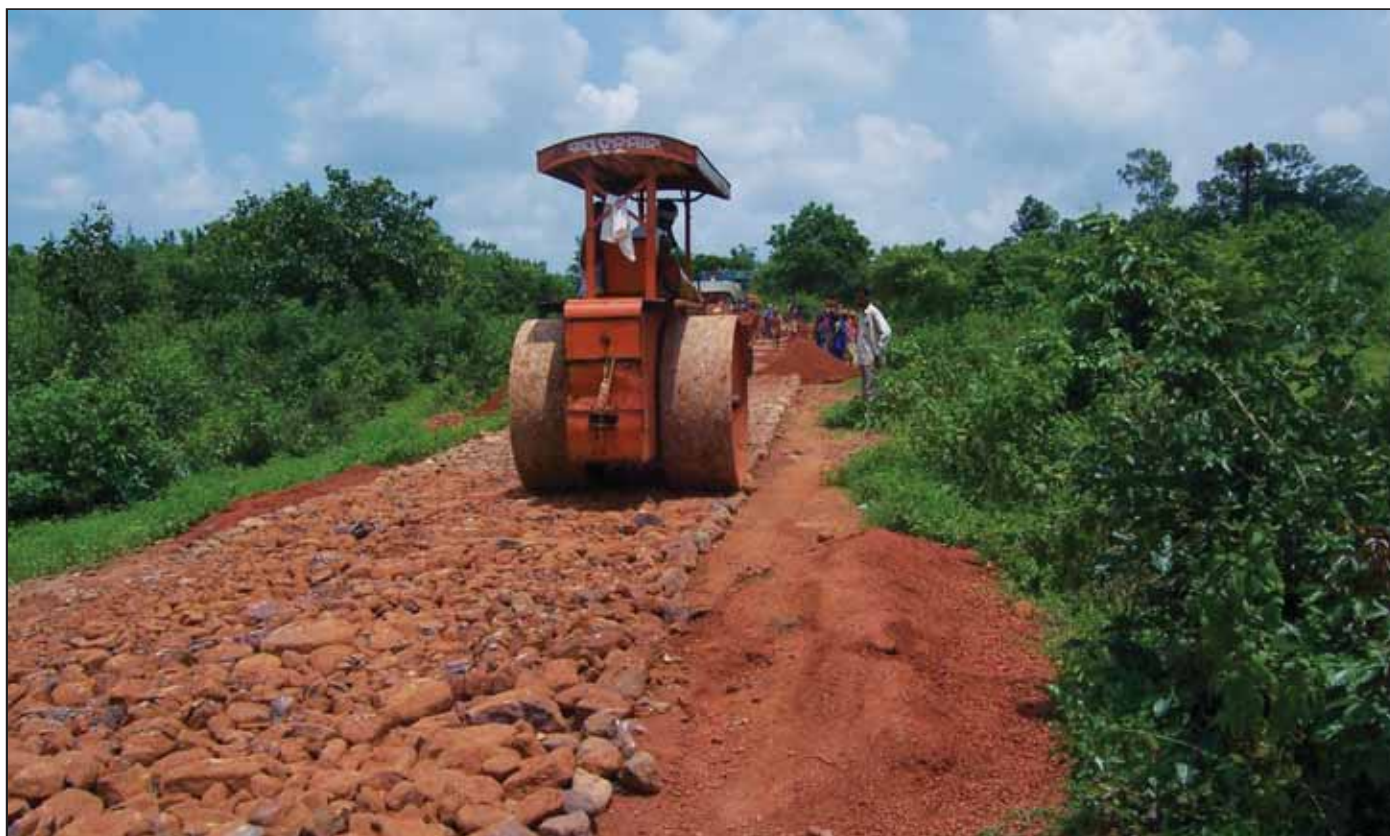
Work in progress under PMGSY
