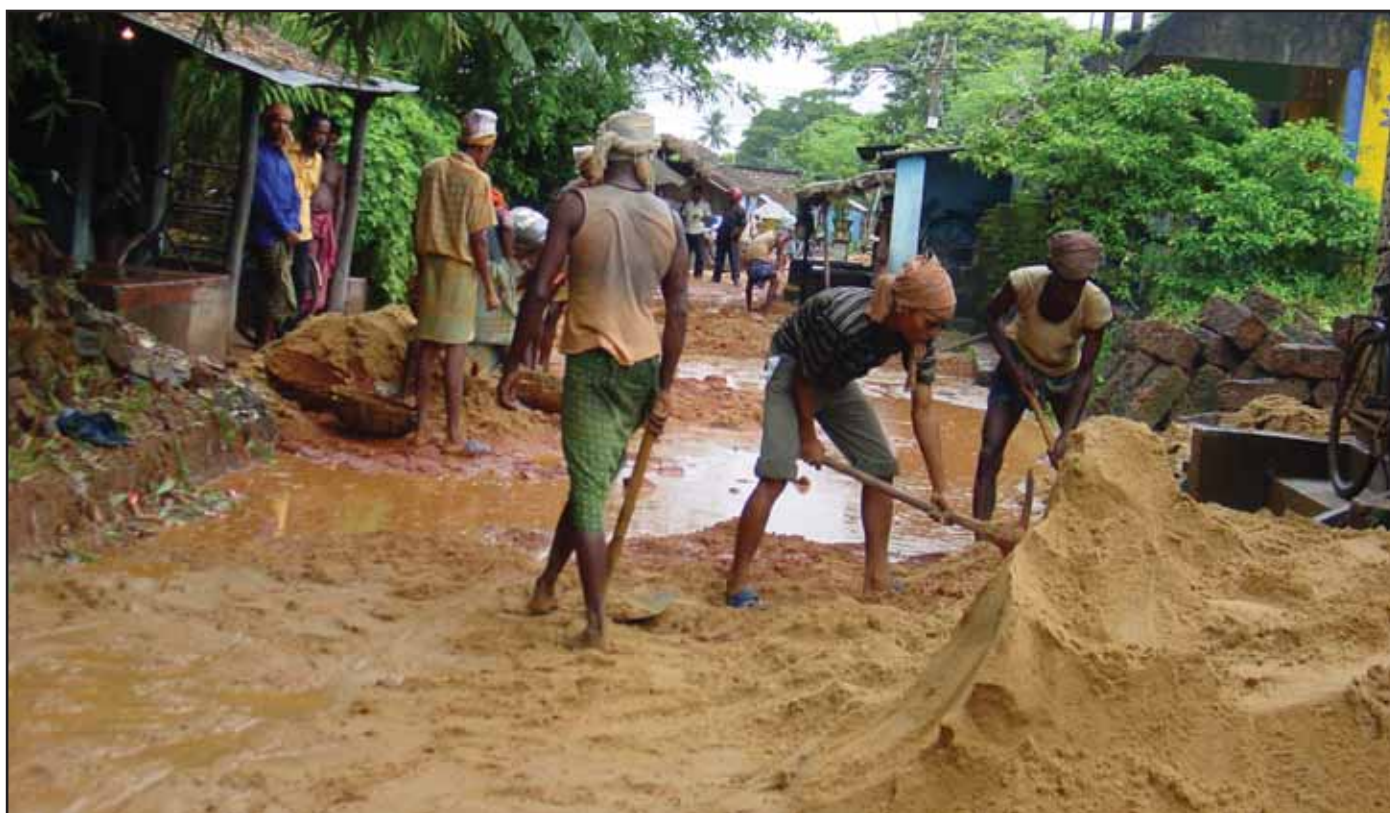
Road construction work in progress under PMGSY
