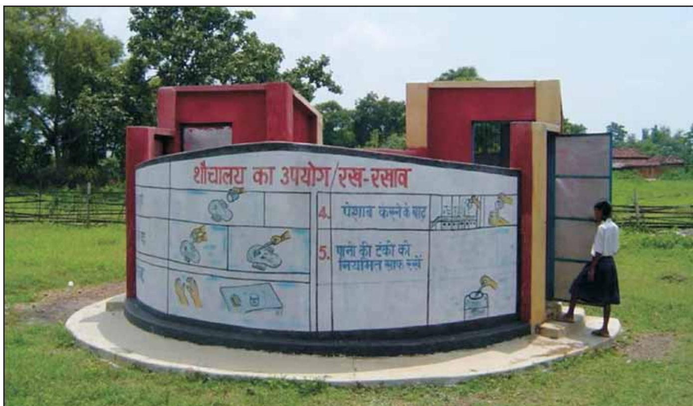
Toilets built under TSC
