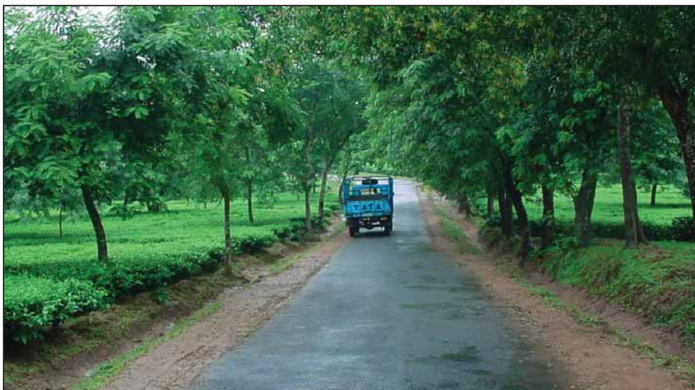
Road constructed under PMGSY providing connectivity between urban & rural areas.
