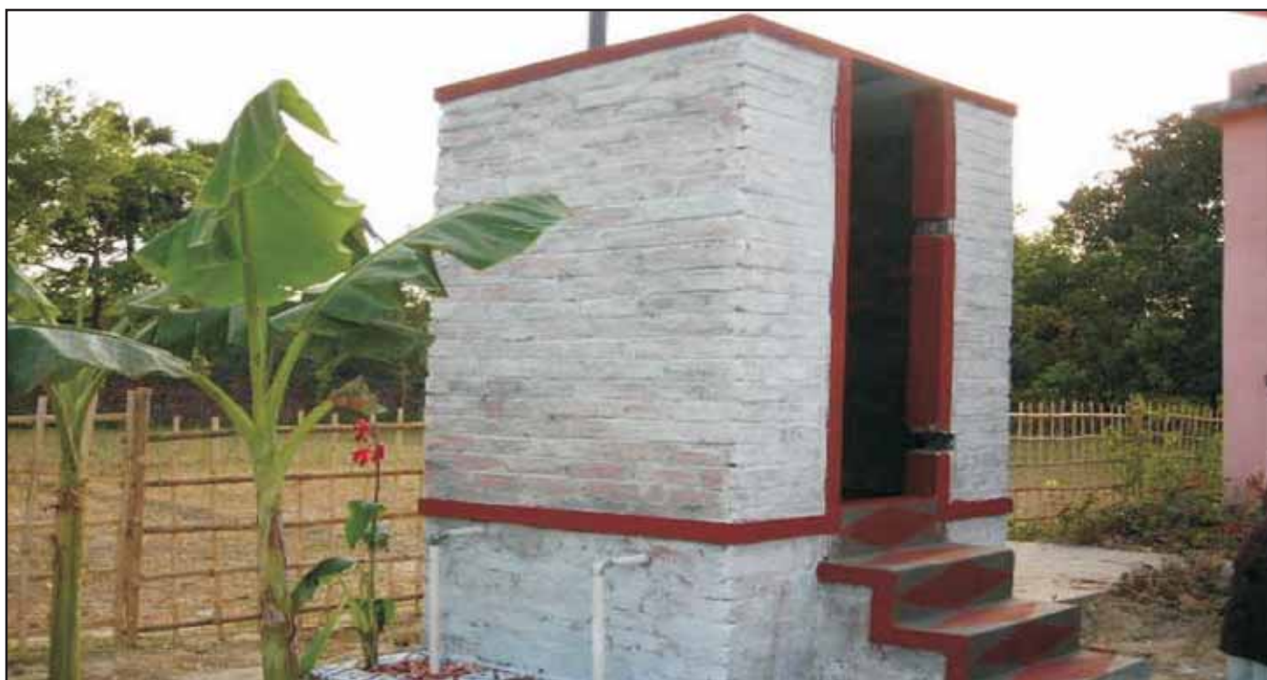
Individual toilets are also part of TSC
