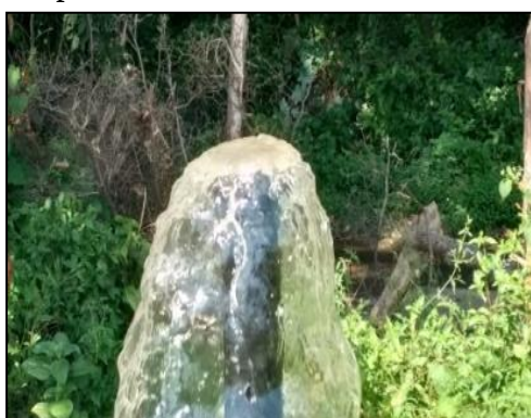
Outlet of pipeline of Subsurface Dam infields
