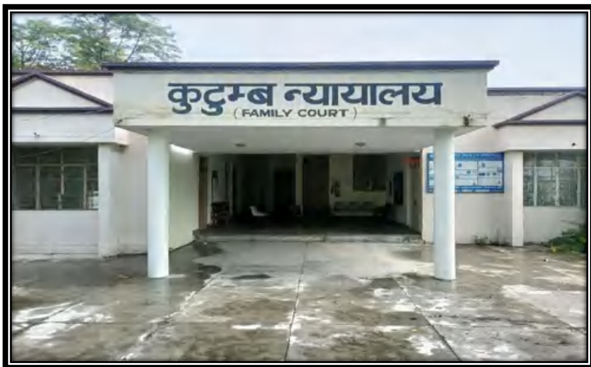
Family Court I Building, Rudrapur, U.S. Nagar
