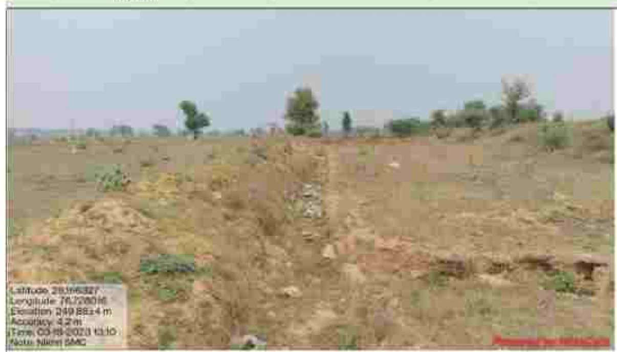
Figure 6.69: Recharge Trench for Soil Moisture Conservation in Masani bandh, Rewari range
