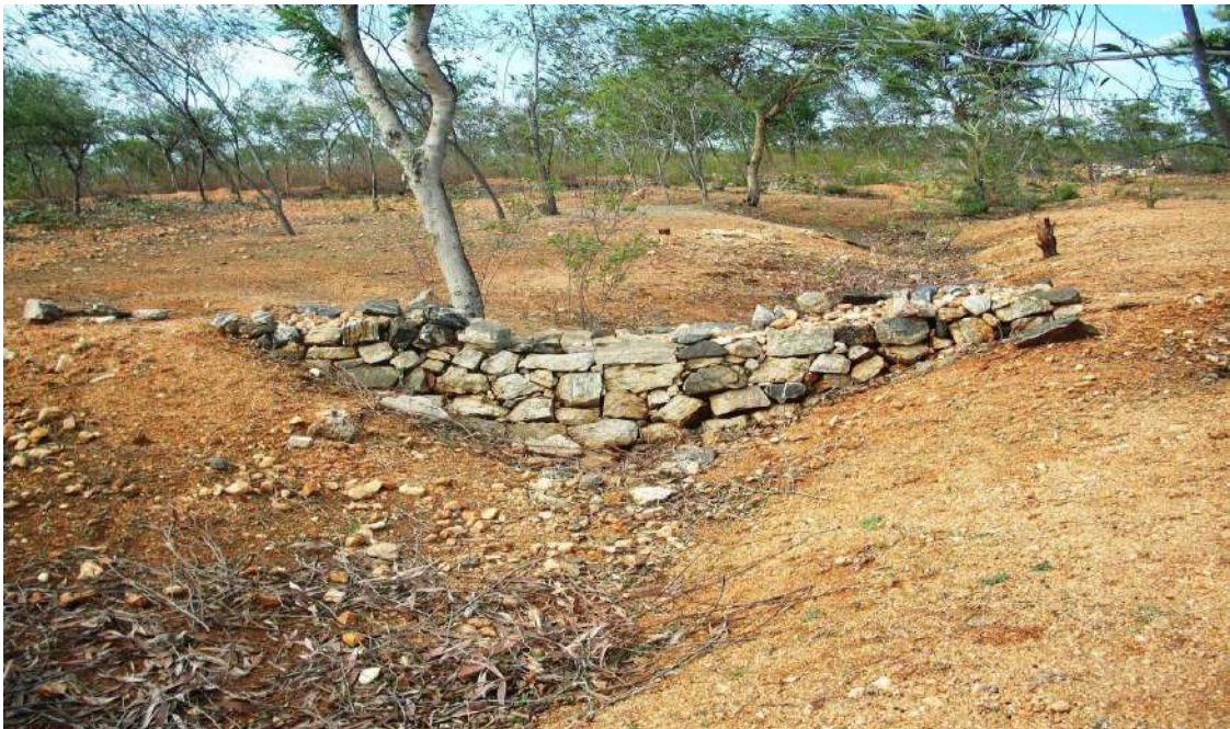
Fig 3.9: Loose Stone Check Dam
