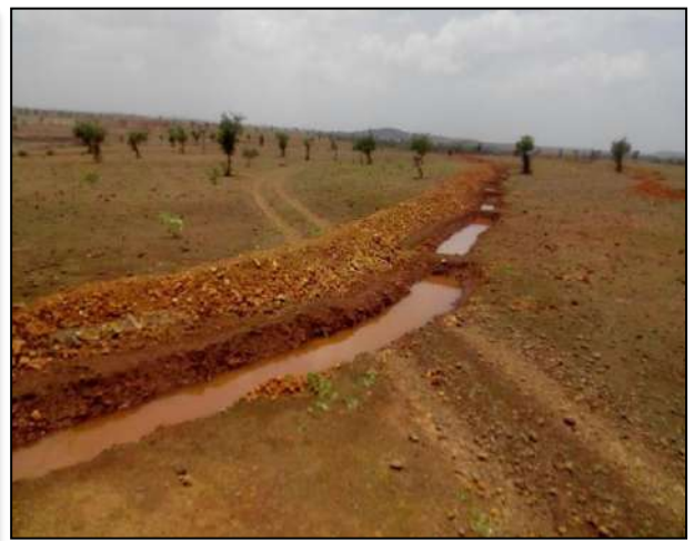
Fig 3.7: Continuous Contour Trenches (CCT)
