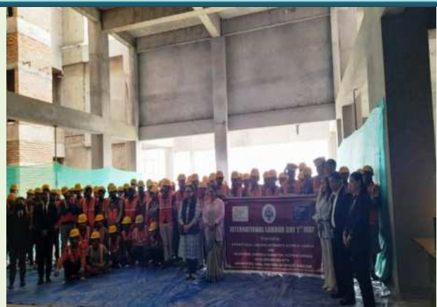
Construction site of New Super Specialty Hospital, Namchi on 29.04.2023
