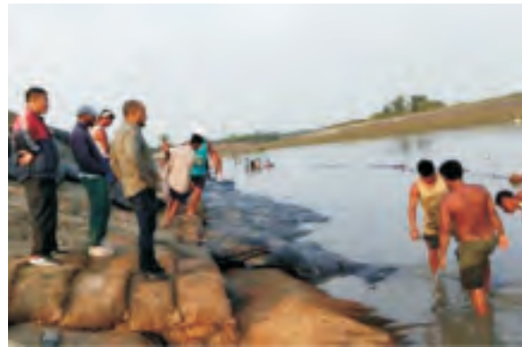
Laying of geo bag filled with earth
