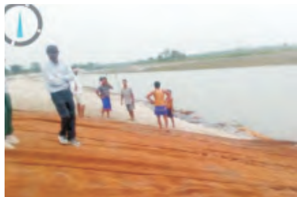
Laying of Coir mat above geobag & coir bag
