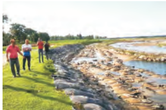
Bank protection work at Bhogdebri area on the Right Bank of River Mansai in Cooch Behar District, West Bengal
