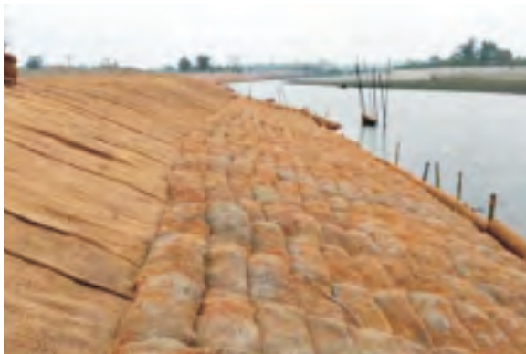
Laying of Coir bag filled with earth
