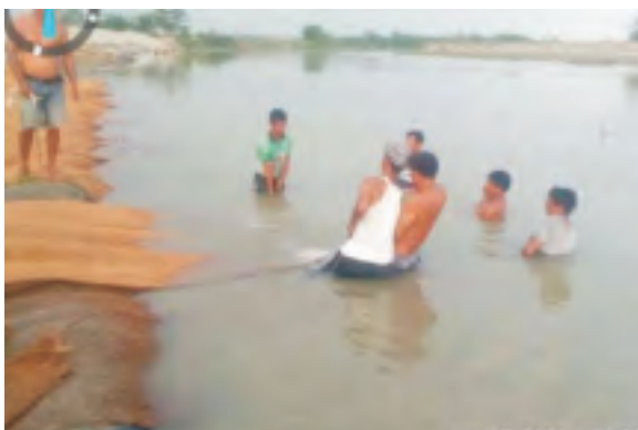
Laying of Coir mat above geo-bag
