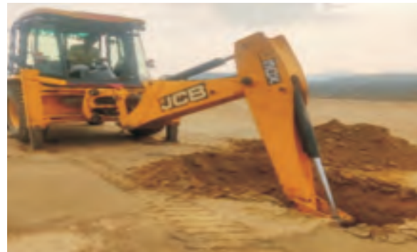
Collection of borrow area Soil samples
