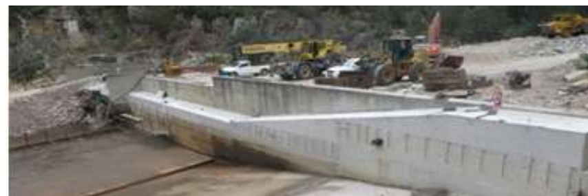
Figure 2. Reconstruction of left flank damaged wall
