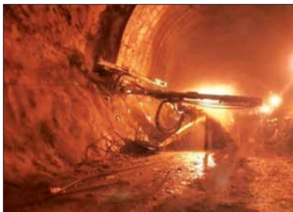
Drilling for Rock Bolt at TRT
