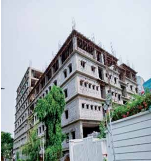
Construction of new building at NRIADD, Salt Lake, Kolkata, West Bengal
