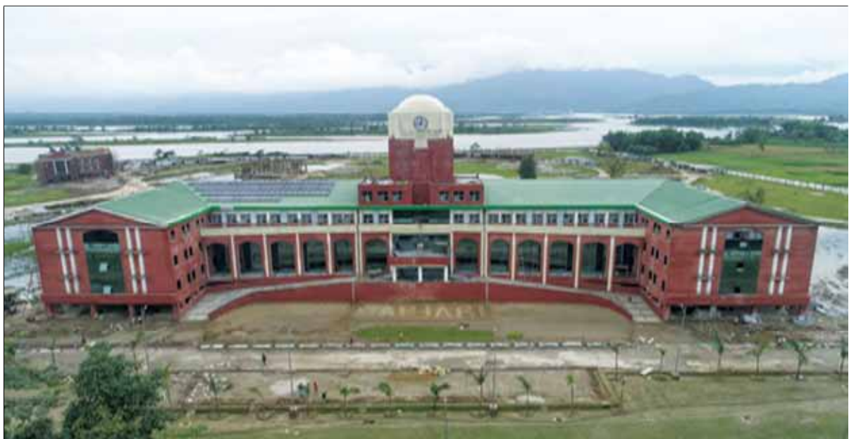
Construction and site development works of IARI at Dhemaji, Assam
