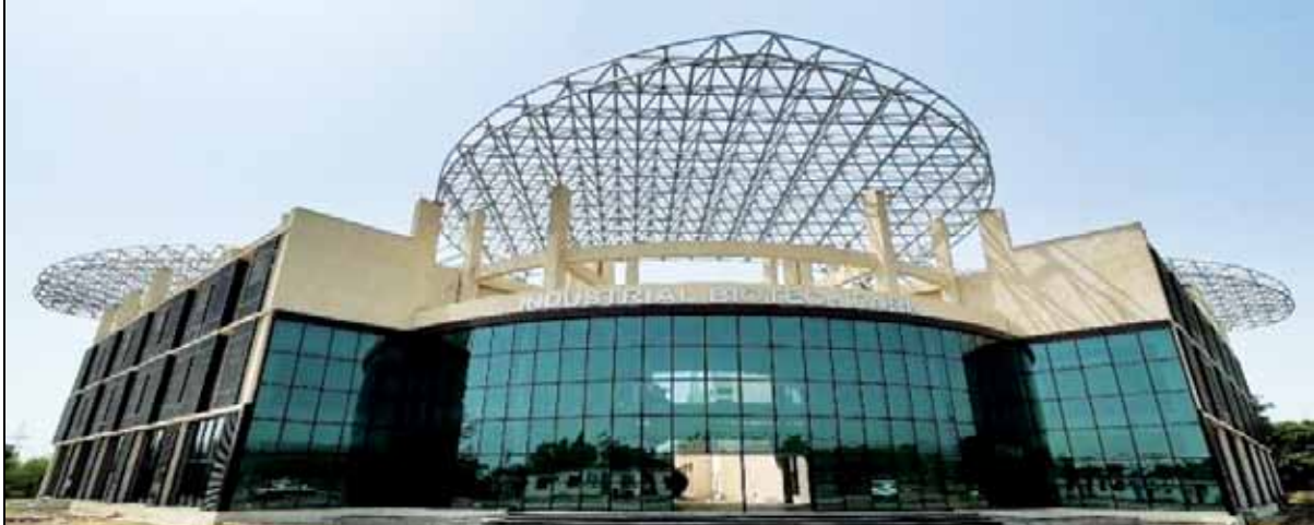
Construction of Industrial Biotech Park at Kathua, Jammu & Kashmir
