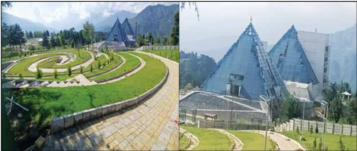
Development of Tourist Facilities at Mantalai, Jammu & Kashmir
