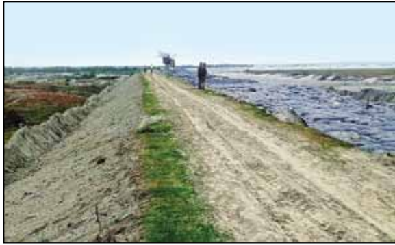
Conversion of Tie-bund into embankment on River Brahmaputra Near Dibrugarh, Assam
