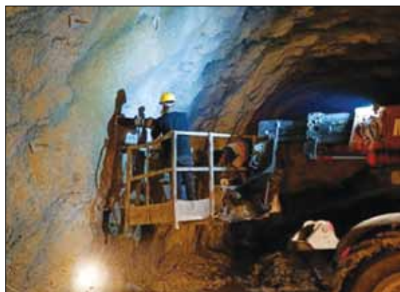
HRT Rock Bolt Testing
