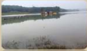
Wet Dredging at Mangalam Dam
