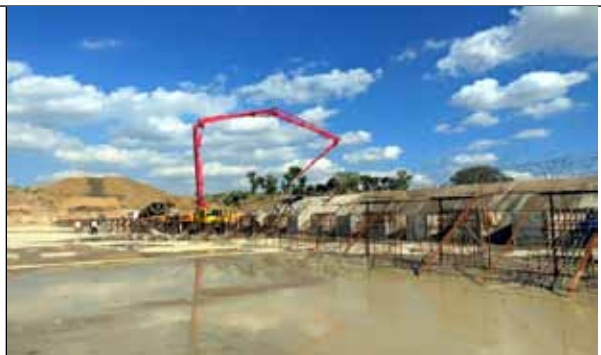
Concreting is in progress by boom placer
