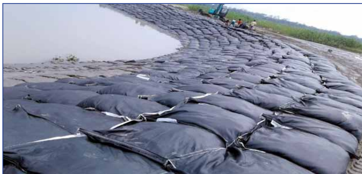
Protection of Majuli Island from flood and erosion of River Brahmaputra (Bankrevetment) at Salmara, Majuli
