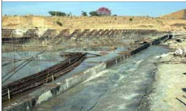
Curing of Spillway Structure by ponding
