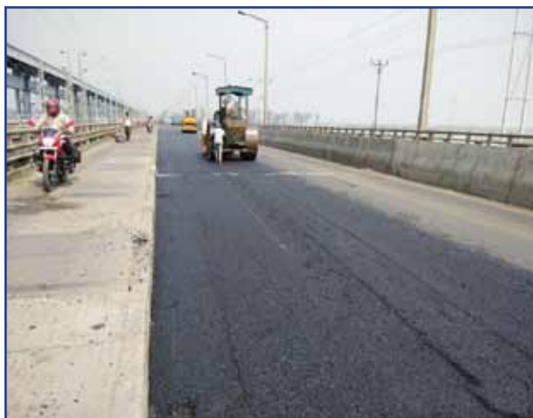
Renovation/Special repair and improvement of PSC bridge road over Farakka Barrage
