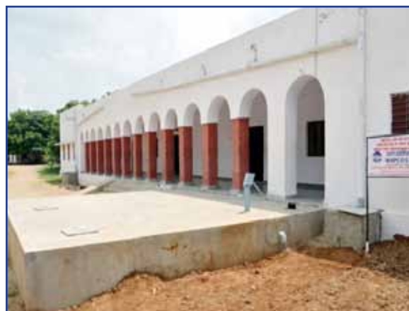
Rain Water Harvesting Tank constructed at Tilonia, Rajasthan
