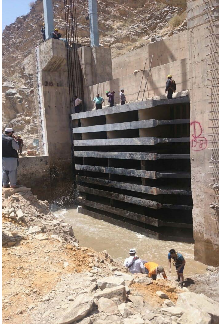
Diversion Tunnel Gate Closure, Salma Dam Project, Afghanistan
