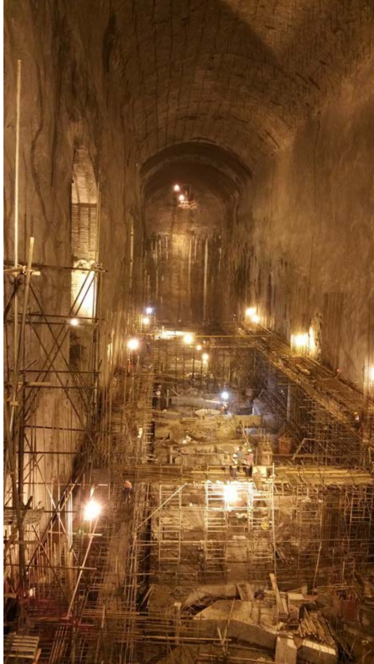
Construction of underground Powerhouse cavern, Punatsangchhu-I Hydro-Electric Project
