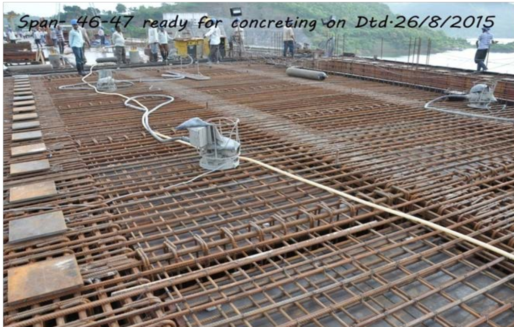
Phase-I construction of Sardar Sarovar Dam-Reinforcement ready for concreting in span 41-42
