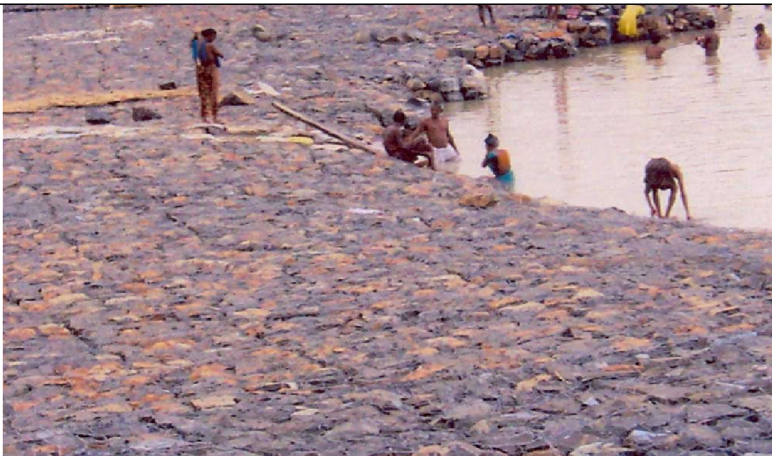
Embarkment pitching along the left bank of River Ganga under the flood protection works
