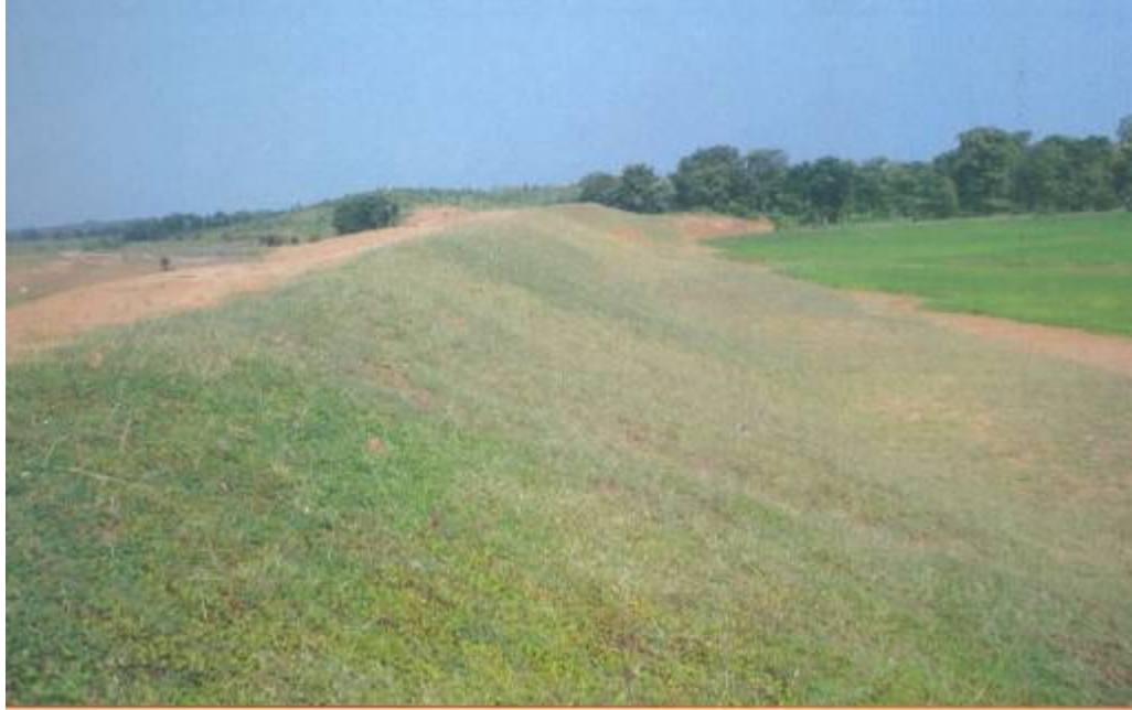
★ Turfing work on left embankment of river Tel
