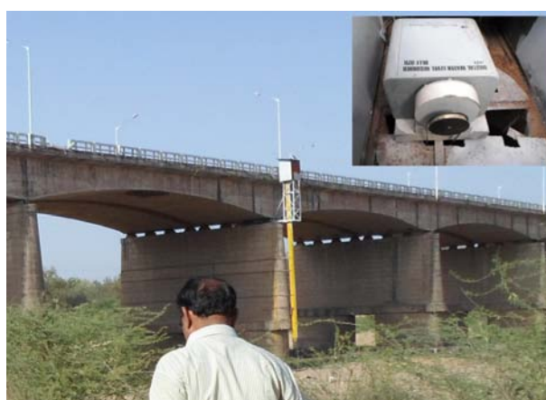
FIG 3.10B: A SHAFT ENCODER INSTALLED ON THE SIDE OF A BRIDGE IN GUJARAT
