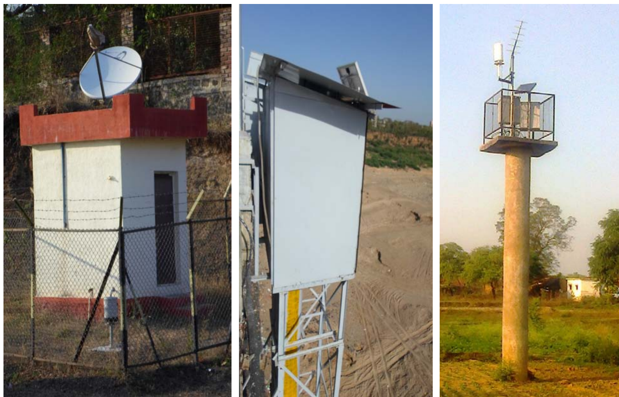
FIGURE 3.16: EXAMPLES OF GAUGE HUTS FOR WATER-LEVEL MONITORING SITES: A) A MASONRY HUT ON A RIVER BANK IN MAHARASHTRA; B) A STEEL ENCLOSURE ON A BRIDGE, GUJARAT; C) A PILLAR ERECTED FOR PROTECTION OF EQUIPMENT BY CWC IN ODISHA
