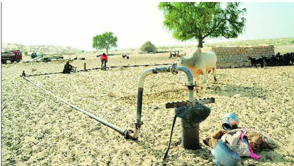
Figure 5.2 A tubewell in the palaeochannels near Tanot, Jaisalmer district, Rajasthan with good quality groundwater (source: http://indianexpress.com/article/india/india-others/finding-an-extinct-river-as-rajasthan-pushes-saraswati-plan-water-marks-all-along-course/ )
