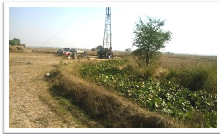
Figure 5.1. Exploratory Drilling by CGWB at Sarswati River Creek/ Channel Reminiscence site at Kurukshetra, Haryana
