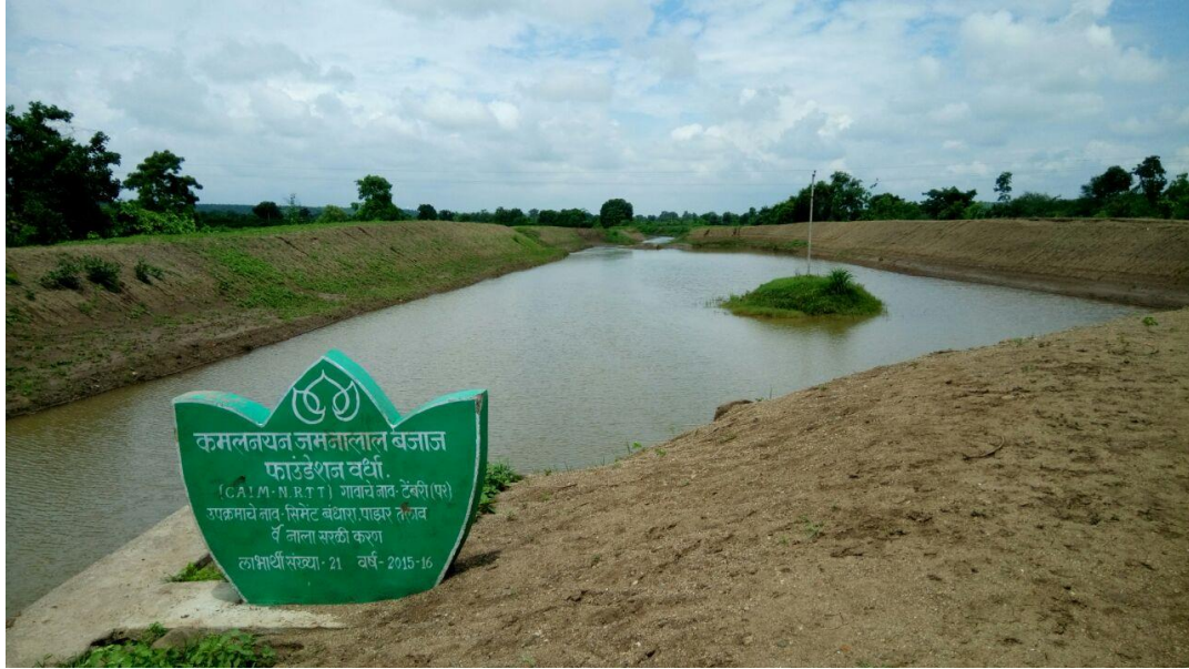
A percolation tank constructed at village Parsodi in Wardha district.
