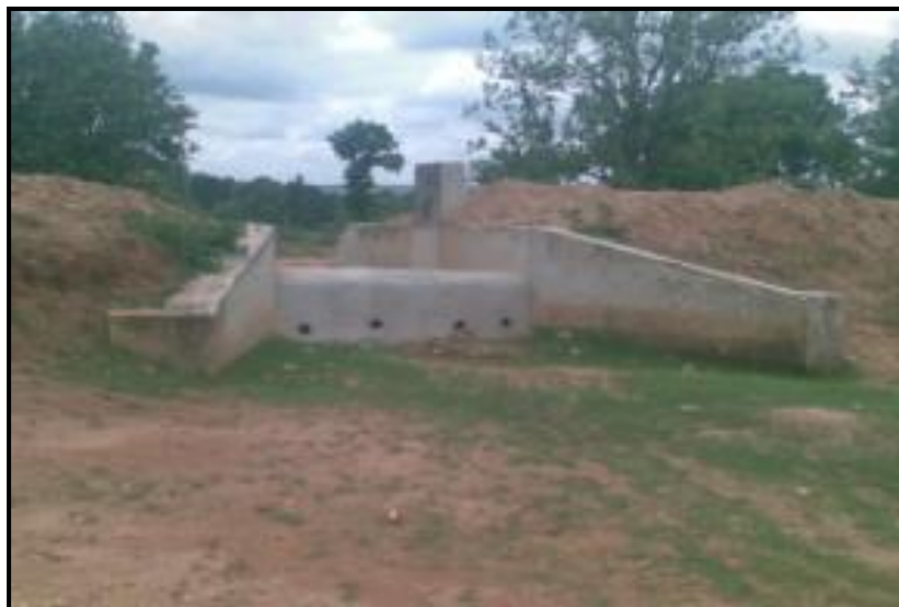
Picture showing the raised spillway
