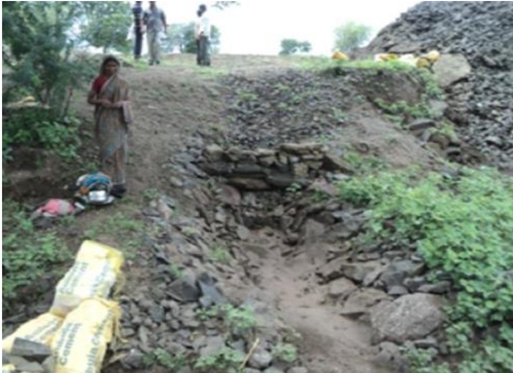
Stabilization Pit for well recharging
