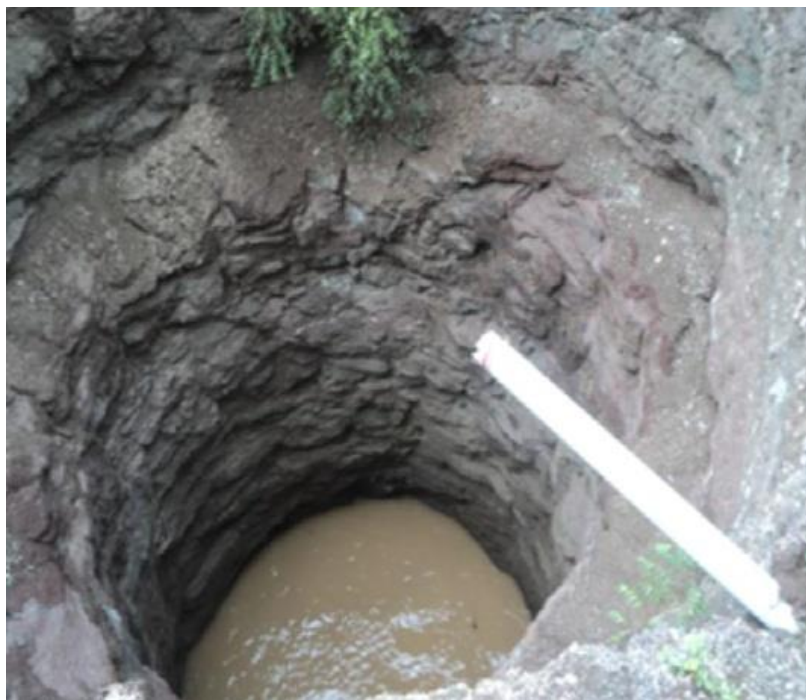
Recharged dug well with inlet pipe
