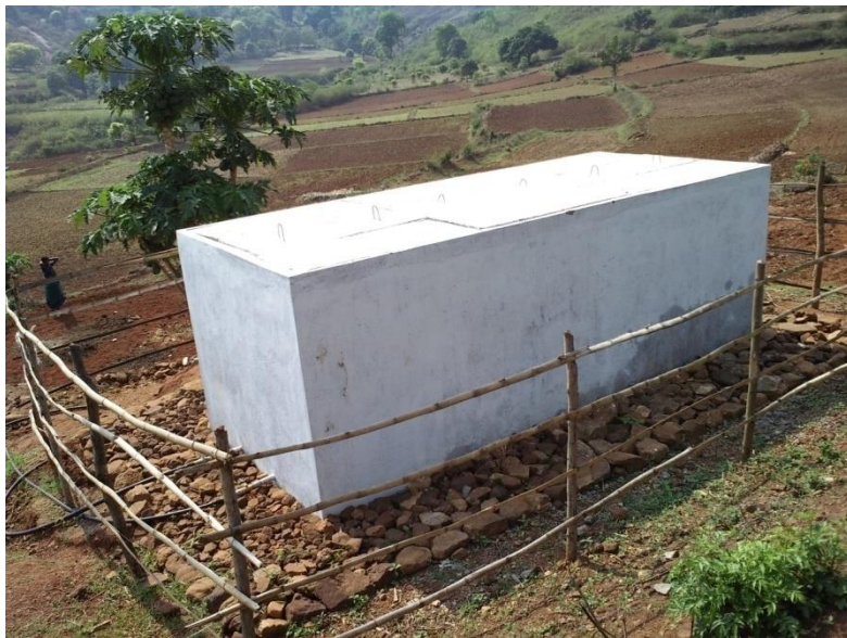
Fully covered top with no contamination
