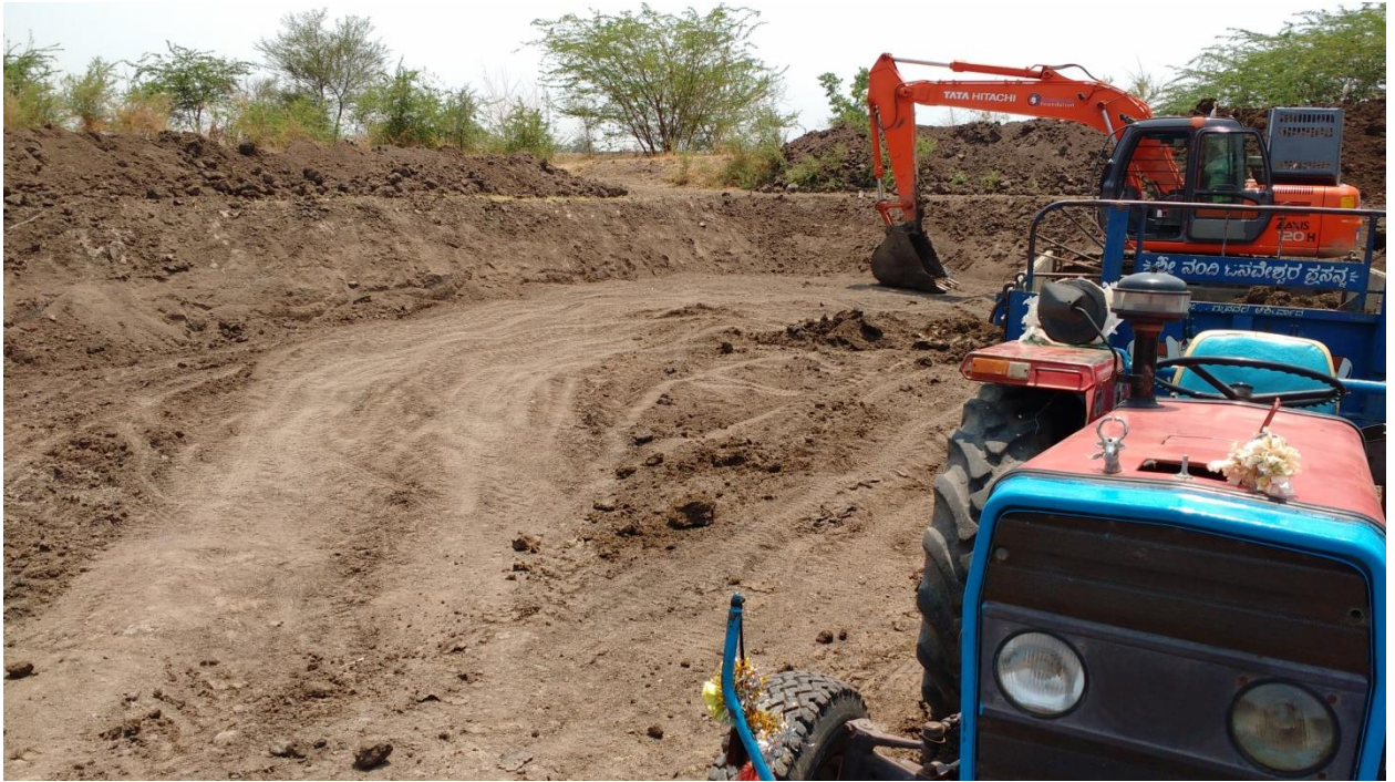
Earthmover at work to dig a farm pond
