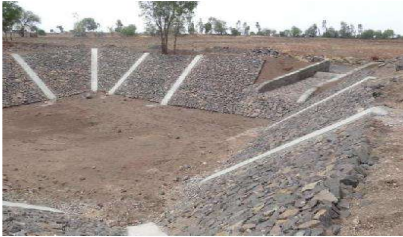
Percolation Pond under construction
