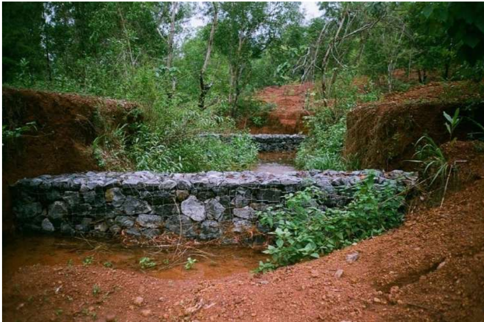
Gabion across a small stream Check Dam across a small stream
