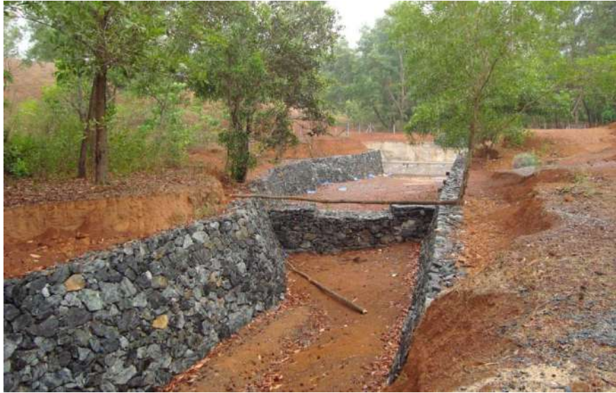
Loose Boulder Check Dam across a small stream
