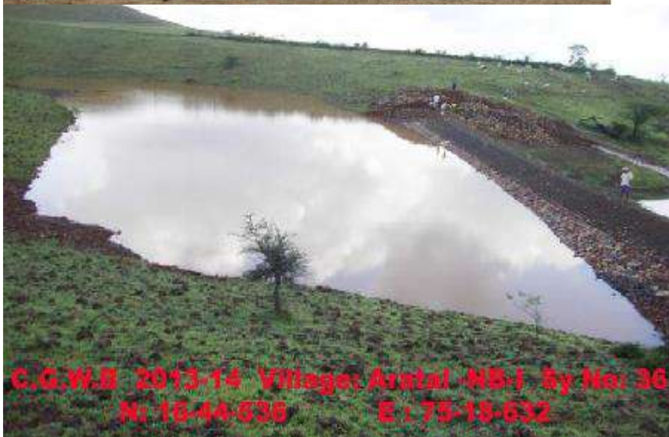
Nala bund constructed in the sub watershed
