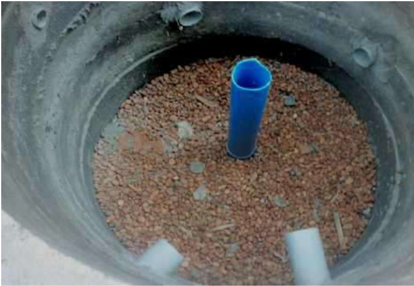
[RECHARGE BORE WELL] OFFICE BUILDING, COLLECTORATE CAMPUS, KHURDA DIST
