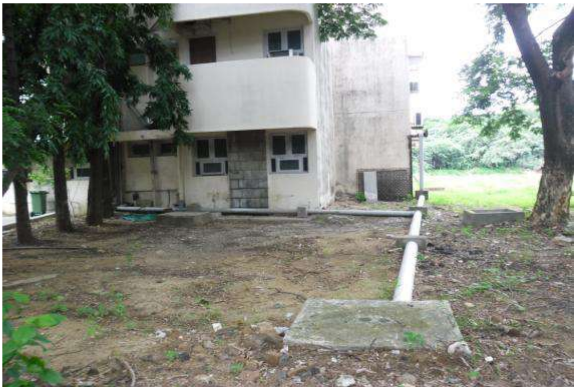
Collection, conveyance and Filtering Unit of roof top rain water harvesting in the premises of the NITTTR, Taramani, Chennai city, Tamil Nadu.
