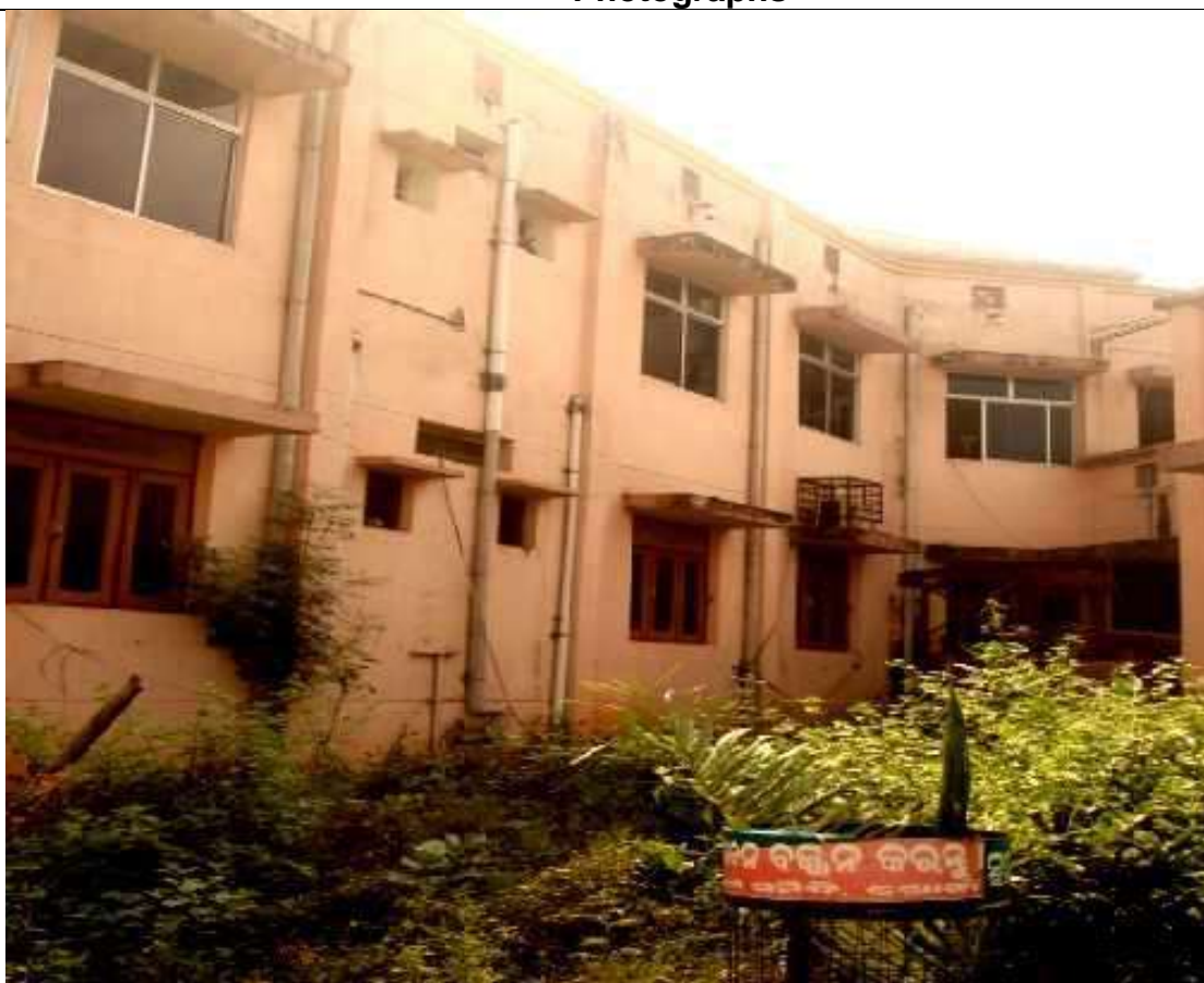
COLLECTION PIPE LINES ON BACK SIDE OF DRDA OFFICE BUILDING, COLLECTORATE CAMPUS, KHURDA DIST.
