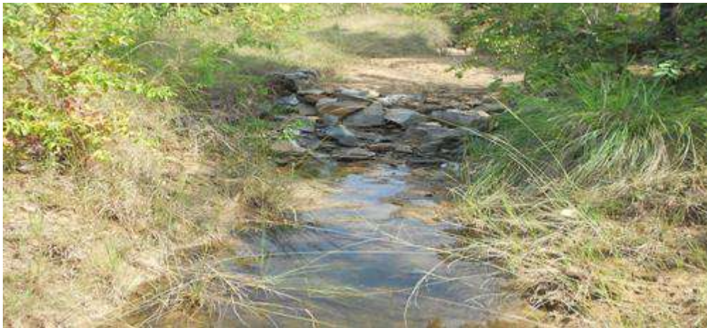
LOOSE BOULDER CHECK DAM--Karmeli mini Watershed , Saintala block, Bolangir dist, Odisha
