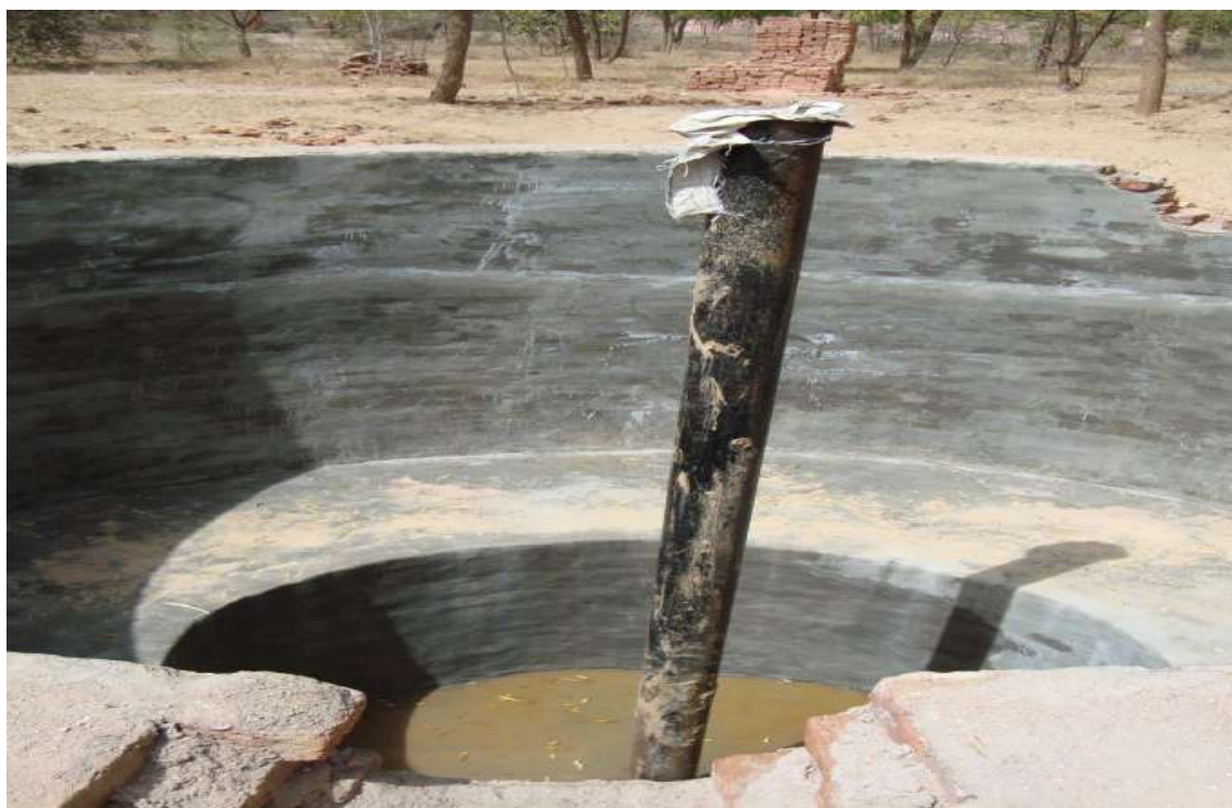
Circular Recharge Pit with filter pit & recharge tube well
