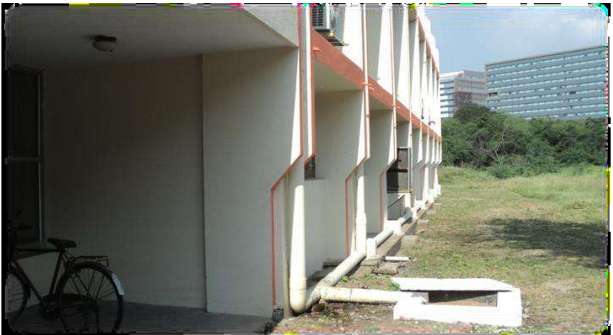
Collection, conveyance and Filtering Unit of roof top rainwater harvesting
