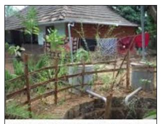
Example of a typical Rooftop RWH Open Well Recharge system, setup under the Mazhapolima program, at a home in Thrissur district.
