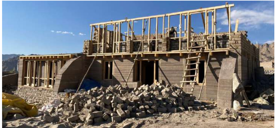
A Rammed earth house under construction in Leh
