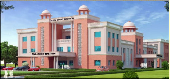
New Civil Court Building Malthon District Sagar
