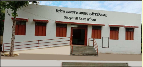
New Civil Court Building, Mandhata (Onkareshwar) District East Nimar Khandwa
