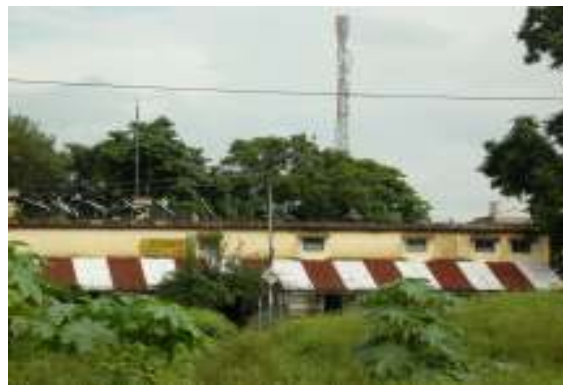
Picture: 1.2 showing railway station of the town Doiwala
