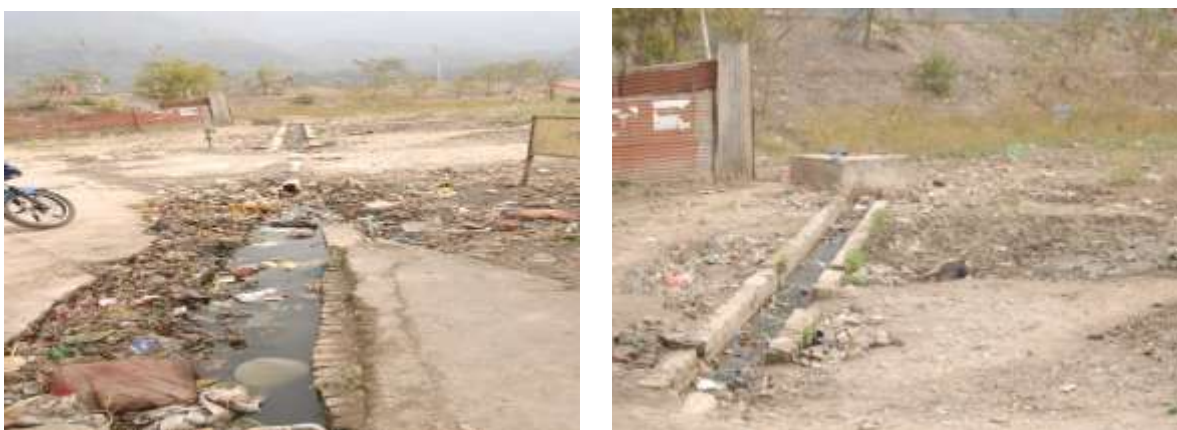
Picture 4.1 showing Existing Scenario of the Drainage System in the Town
