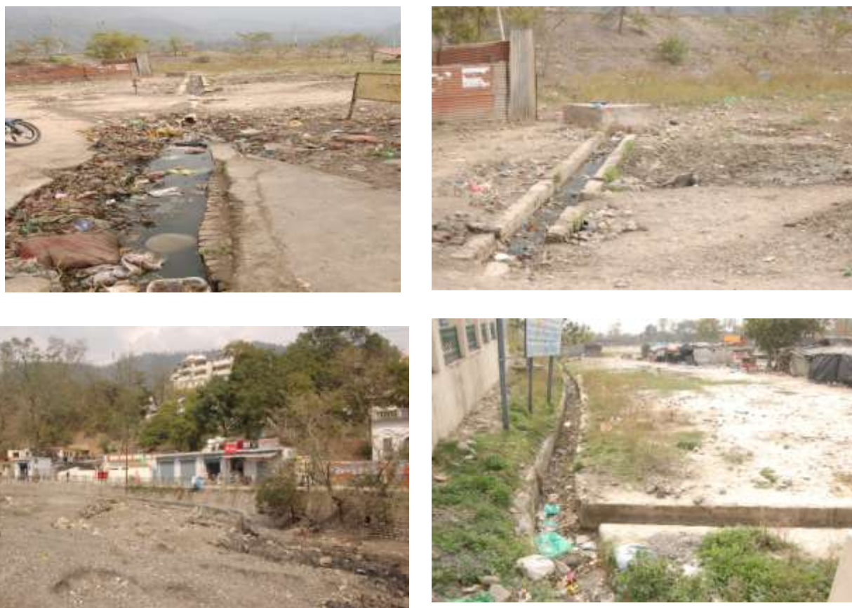
Pictures 3.1 showing drainage problem of the town Muni ki Reti
