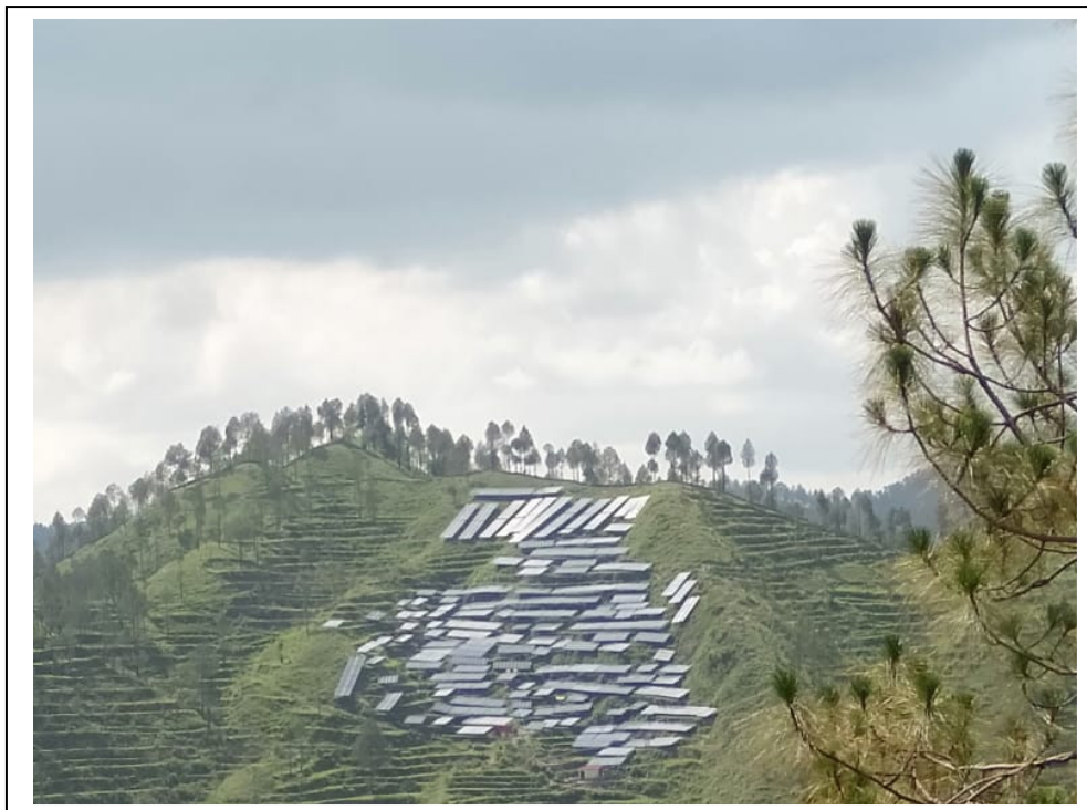
M/s Chandra Shekhar Singh Negi 600 KW Solar Power Plant at Vill-Uregi, Patti-Paidulsyun, Block & Tehsil-Pauri Distt. Pauri Garhwal, Uttarakhand Project Cost: 304.58 Lakh Employment: 4 persons
