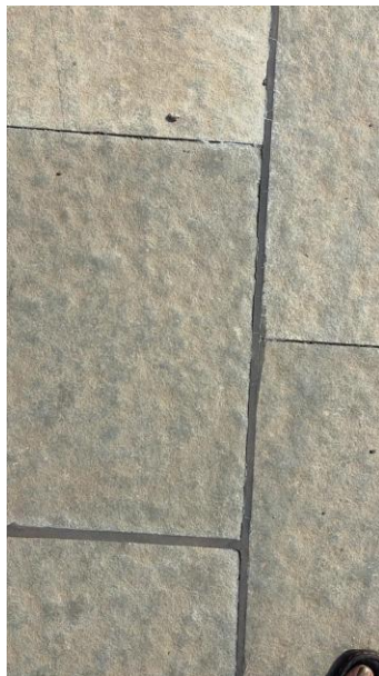
Figure 3: Existing Kota stone – close-up view
