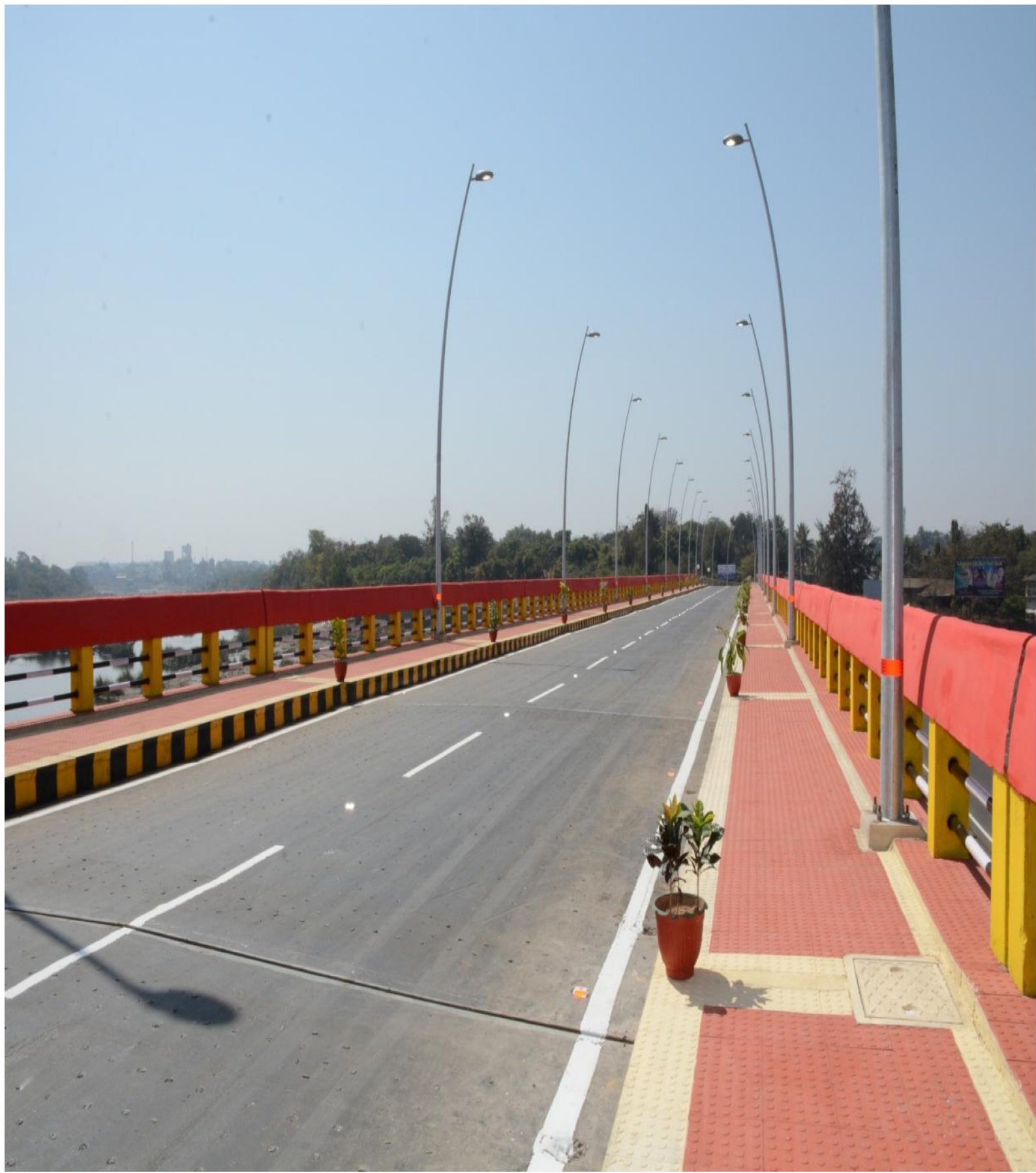
Bridge on Kolak river connecting Daman and Udwada of Gujarat State
